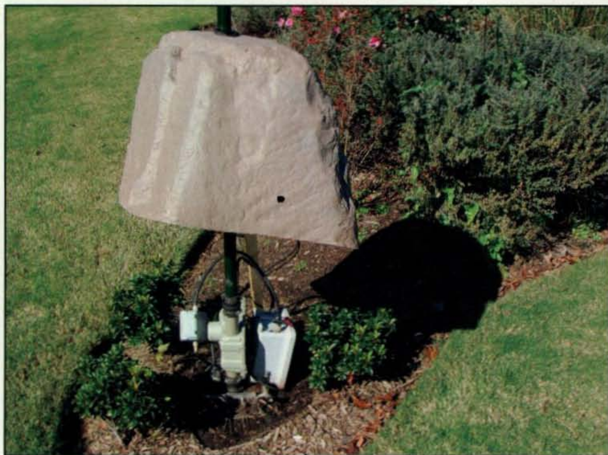
Photo F— Bob raised the "magic rock" (note shadow) to show us the hidden goodies: the radial connection plate, SteppIR motor and mount assembly, coil and relay switch box, and box-protected unun to prevent RF radiation from the coax feedline. Note the cables disappearing into the buried PVC pipe that is routed to his house. (Photo courtesy of KZ5R)
