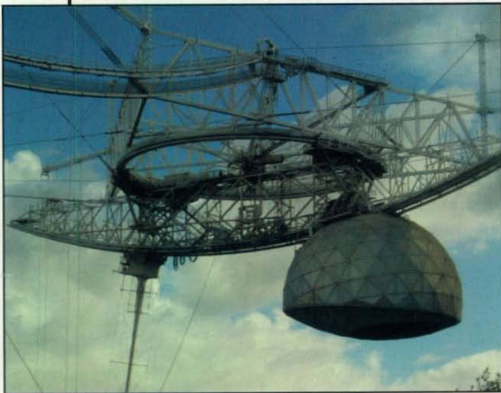
Photo 1—Feed assembly of the Arecibo dish. (W5IU photo)
