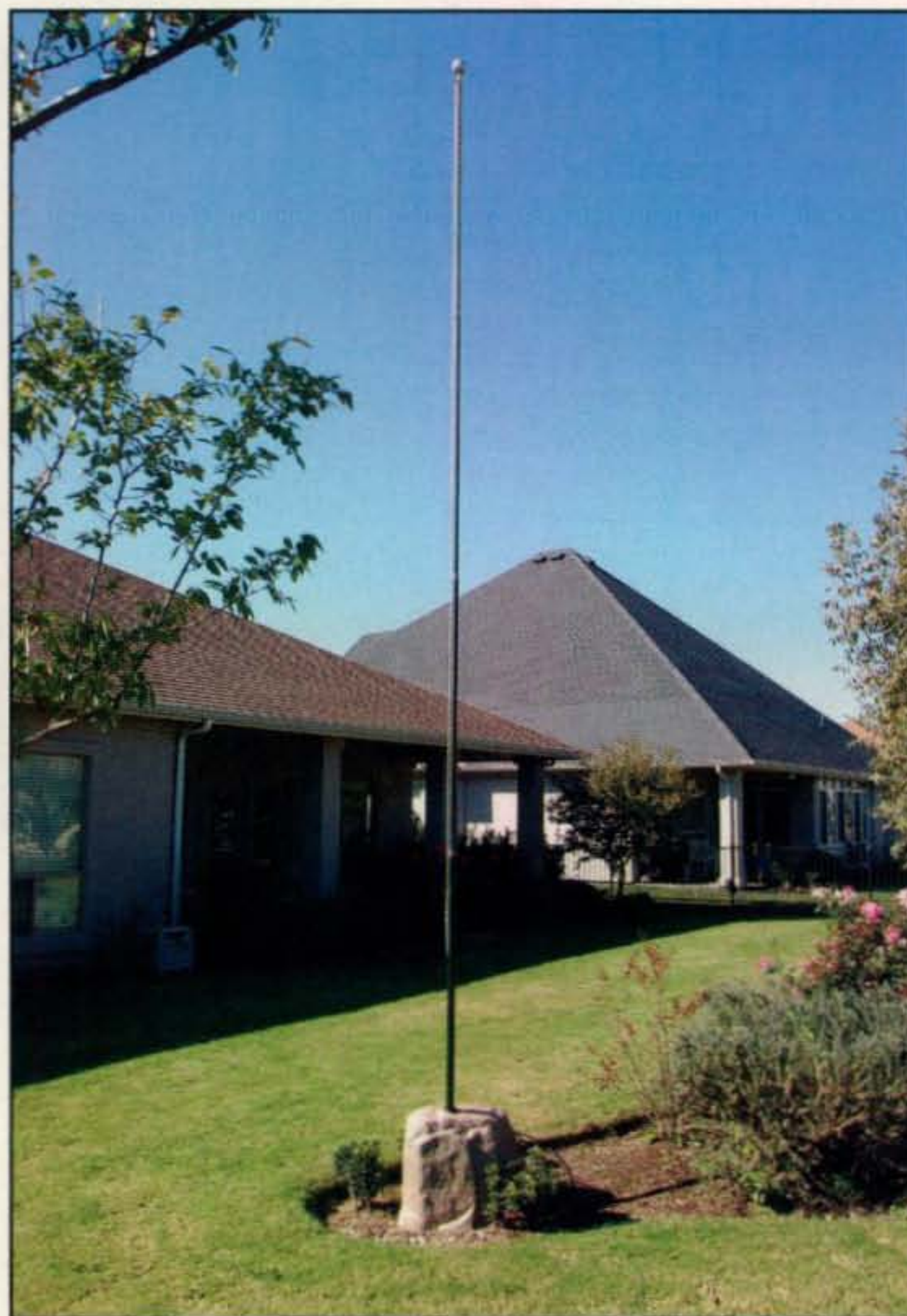
Photo E— The flagpole disguised SteppIR 17-foot vertical with "magic rock" base at the QTH of Bob Rumsey, KZ5R. Bob added a relay-switched base loading coil so the antenna works 40 through 10 meters. It is installed in a clear area for good signal radiation. The hollow "magic rock" was acquired from < www.dekorraproducts.com >. (Photo courtesy of Bob, KZ5R)
