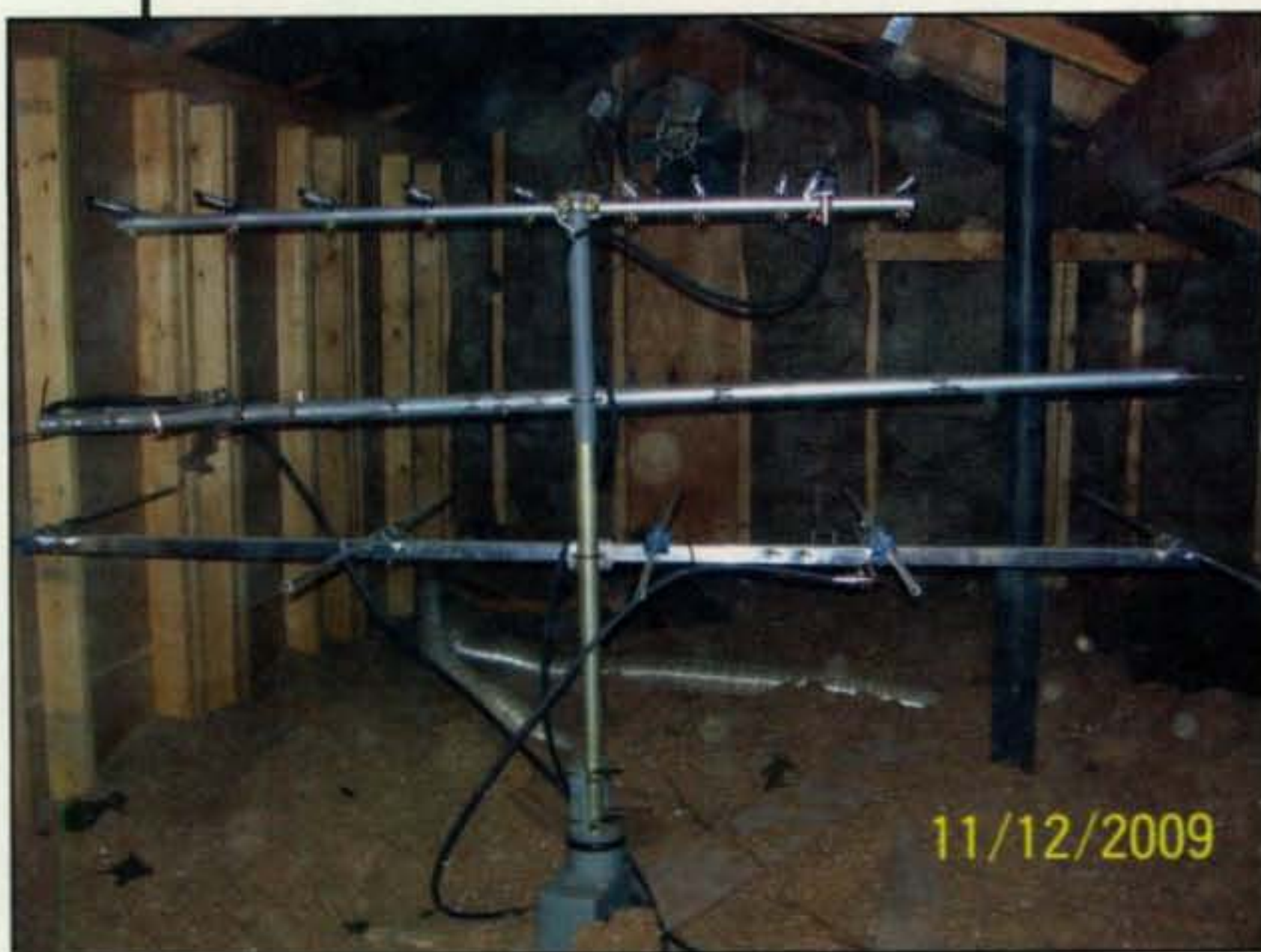
Photo A—A peek in the dark attic of Terry Duehr, KC0VFO, reveals horizontally polarized 2-meter, 70-cm, and 220-MHz Yagis on a rotor-controlled mast attached to the attic floor. The fan on back wall keeps antennas nice and comfy. (Photo courtesy of Terry, KC0VFO)
