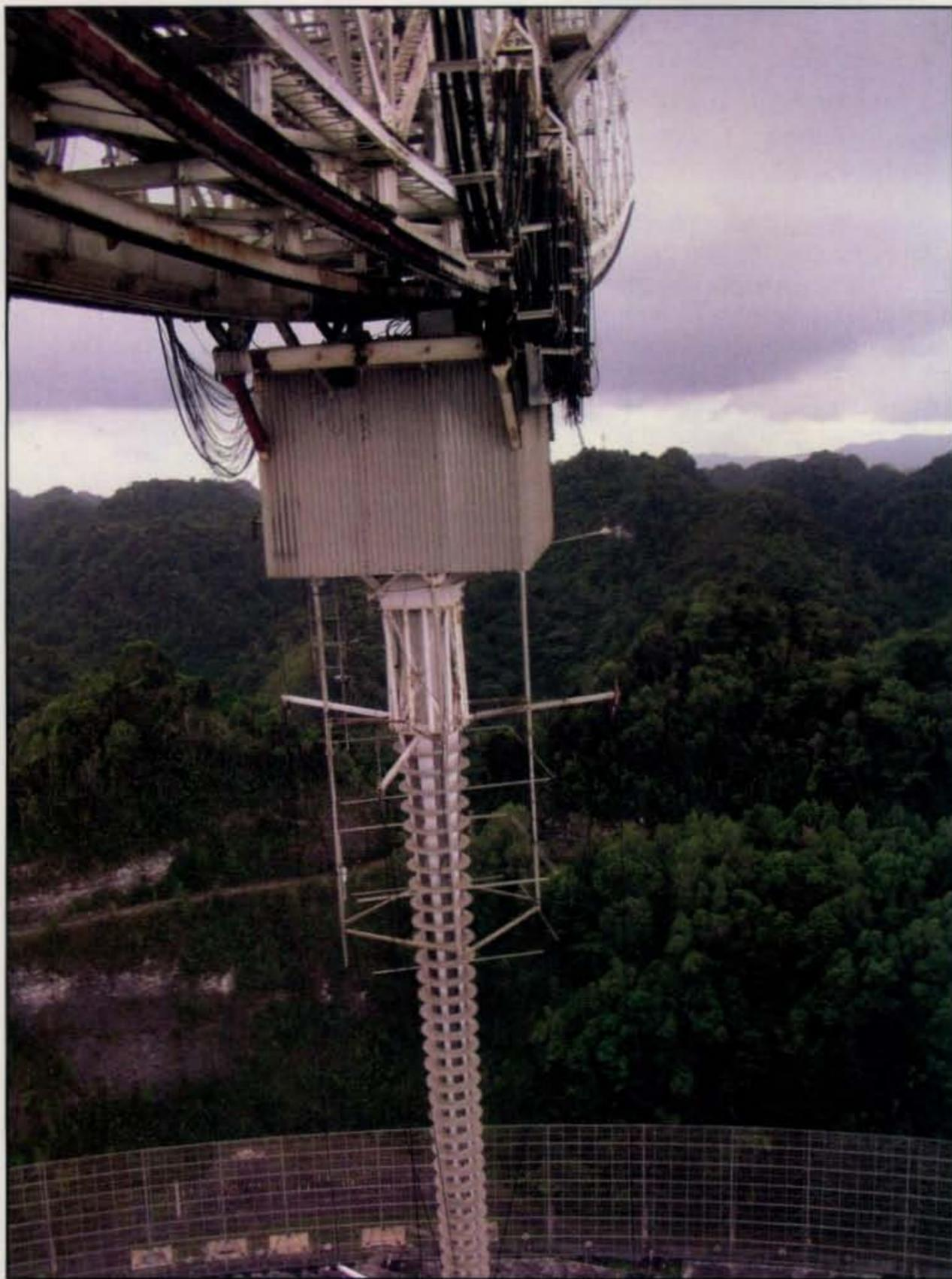
The 432 linear phased array antenna at Arecibo, which efficiently illuminated the 1000-ft. spherical dish surface and collected the linearly aligned received signal images from the dish off the moon. (Photo courtesy of AA6EG)
