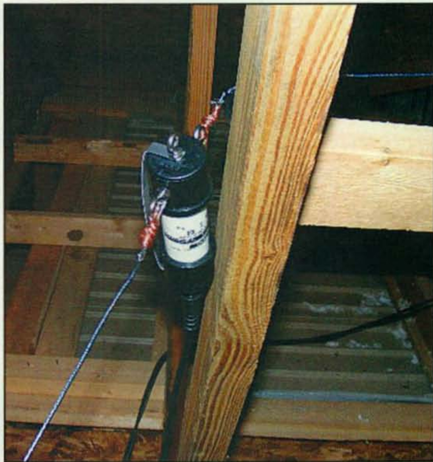
The attic dipole uses insulated copper wire and a 1:1 balun as the center insulator.
