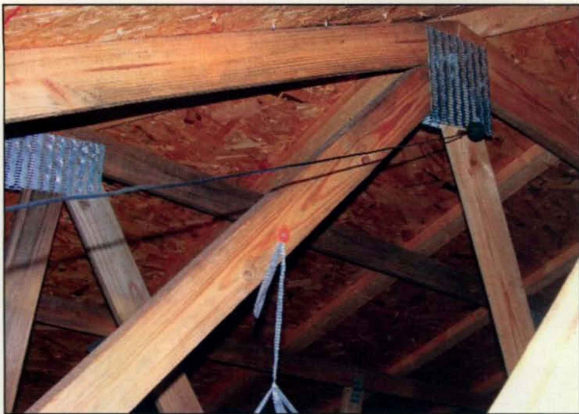
Plastic "egg" insulators secure the ends of the dipole, which kind of snakes its way through the author's attic.
