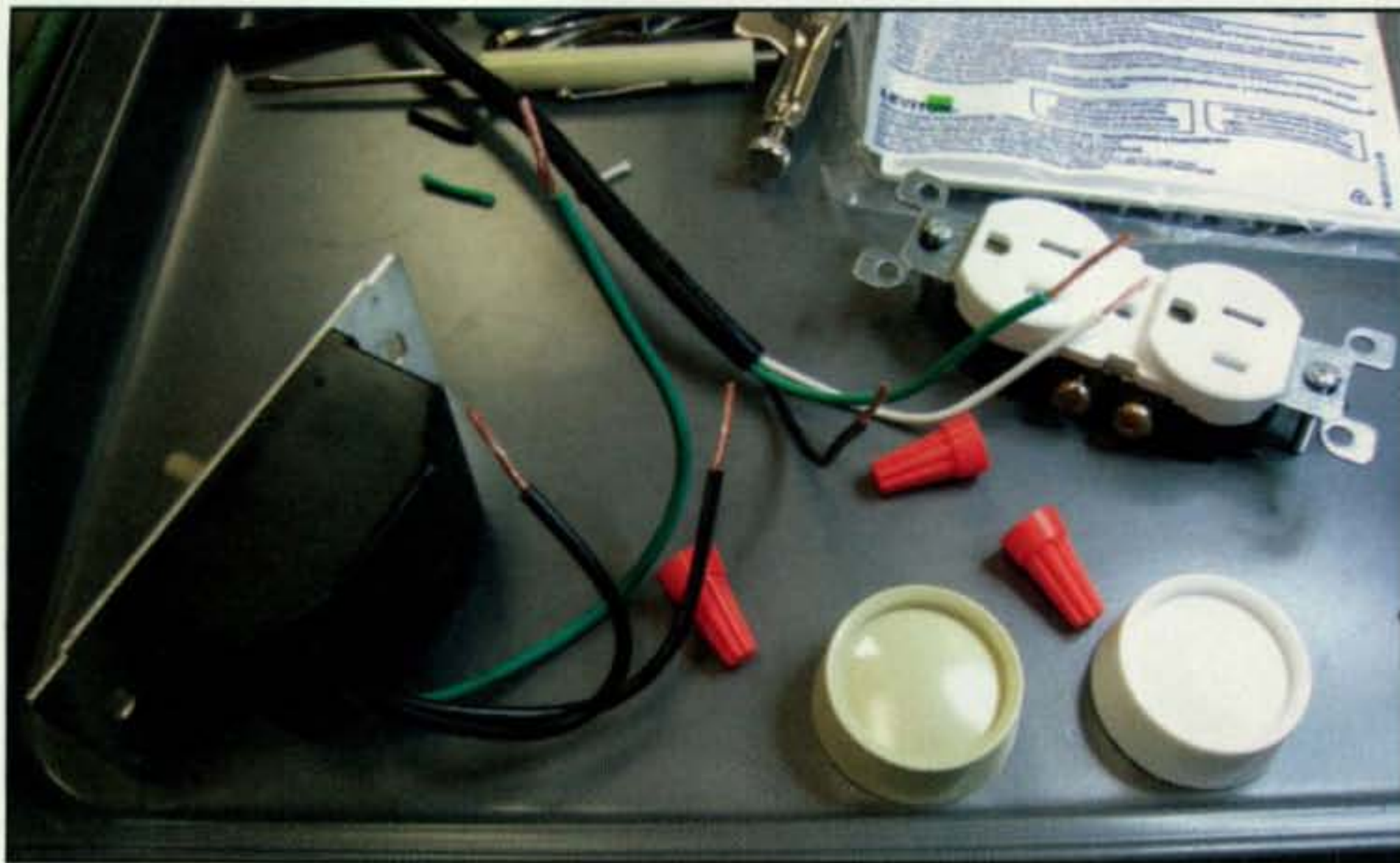
The dimmer and the outlet with wires prepared.
