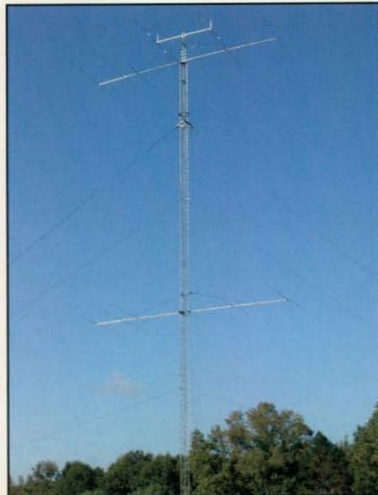
This clean stack of 6-element monobanders helped John, KK9A, set a new North America record in SO20 HP.
