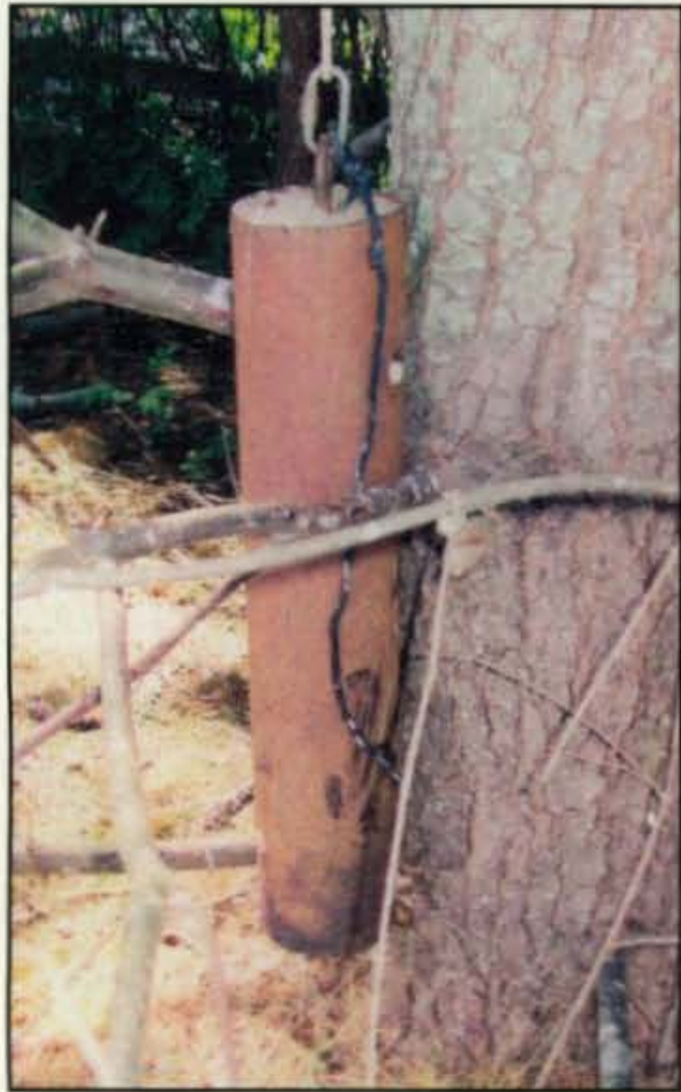
Photo D— Antenna counterbalance. This protects the support ropes from wearing and breaking due to wind.
