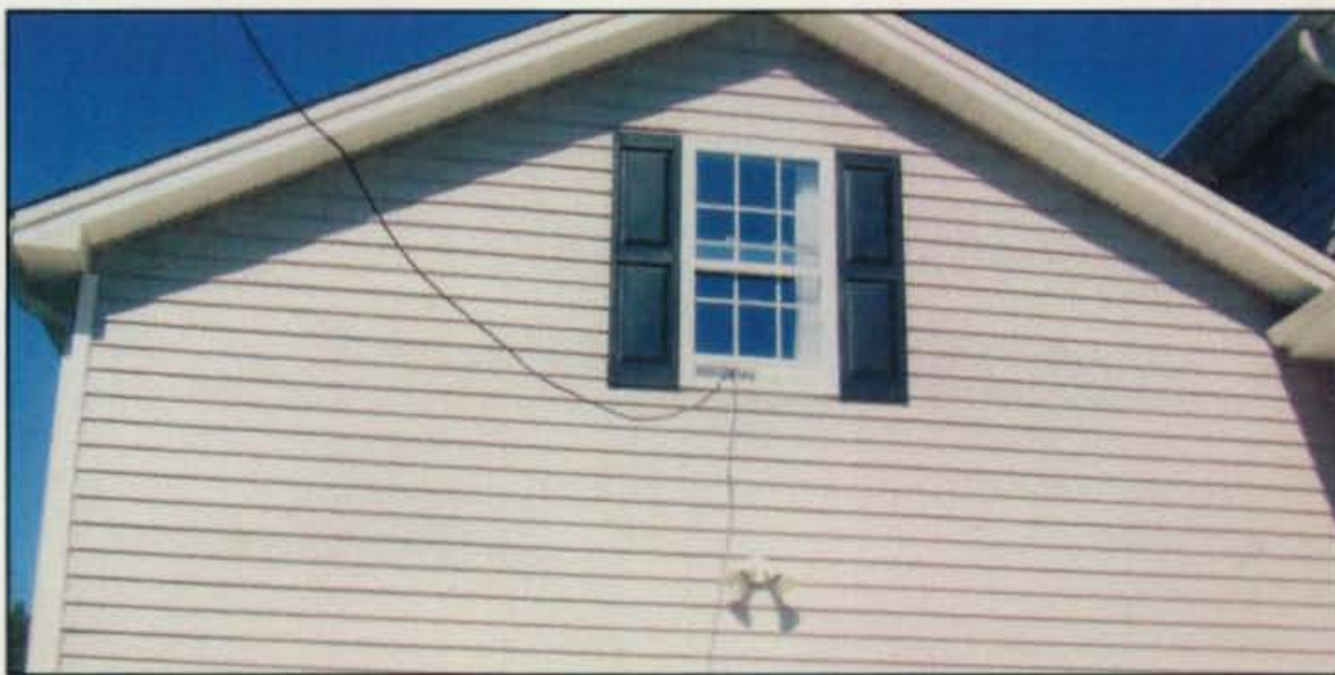
Photo C— Transmission line to feed-through panel in "bonus room" (attic) window.
