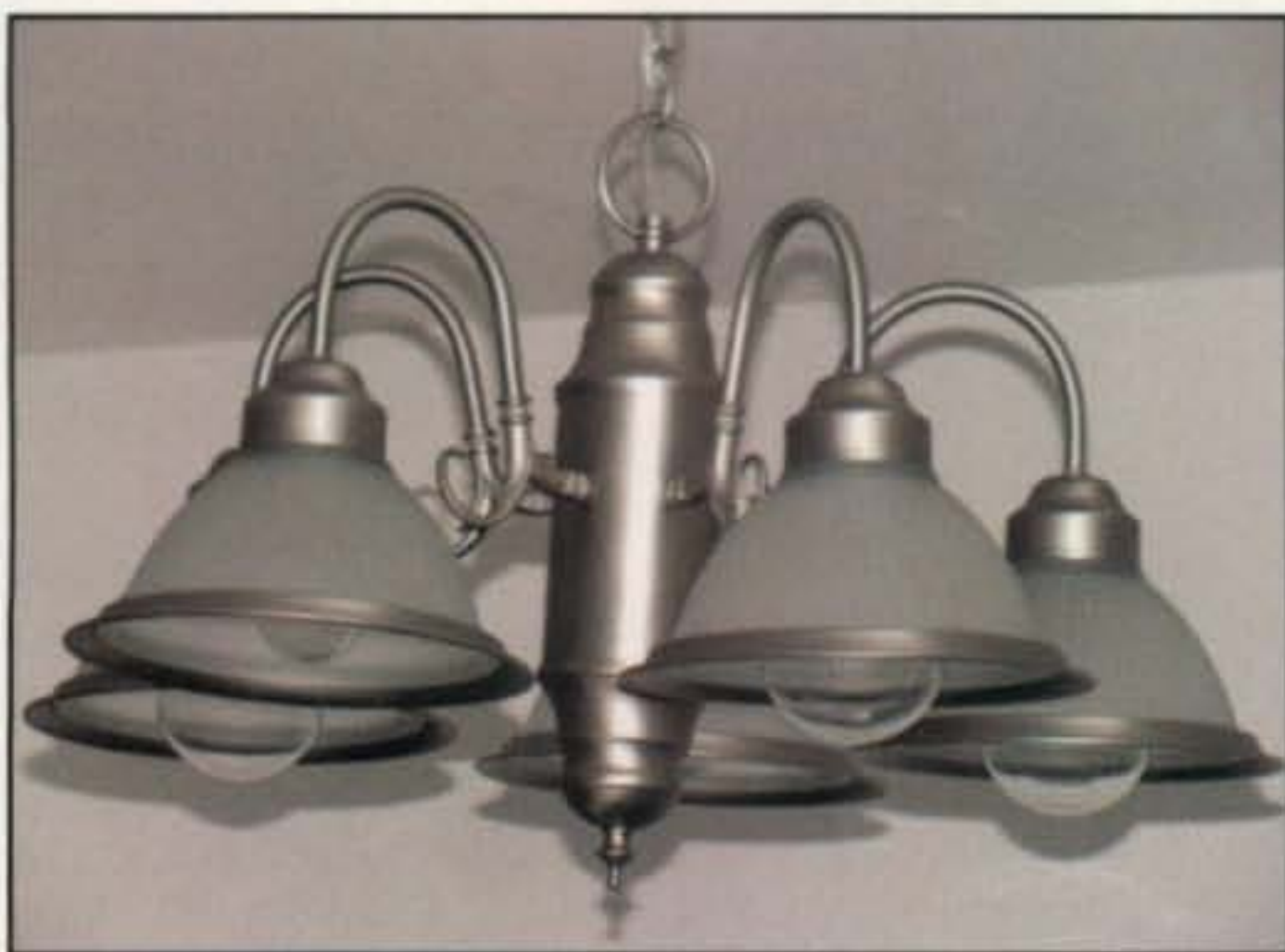
Photo C— These low-wattage incandescent bulbs with clear-glass envelopes are also very good and may be better than either CFLs or LEDs.
