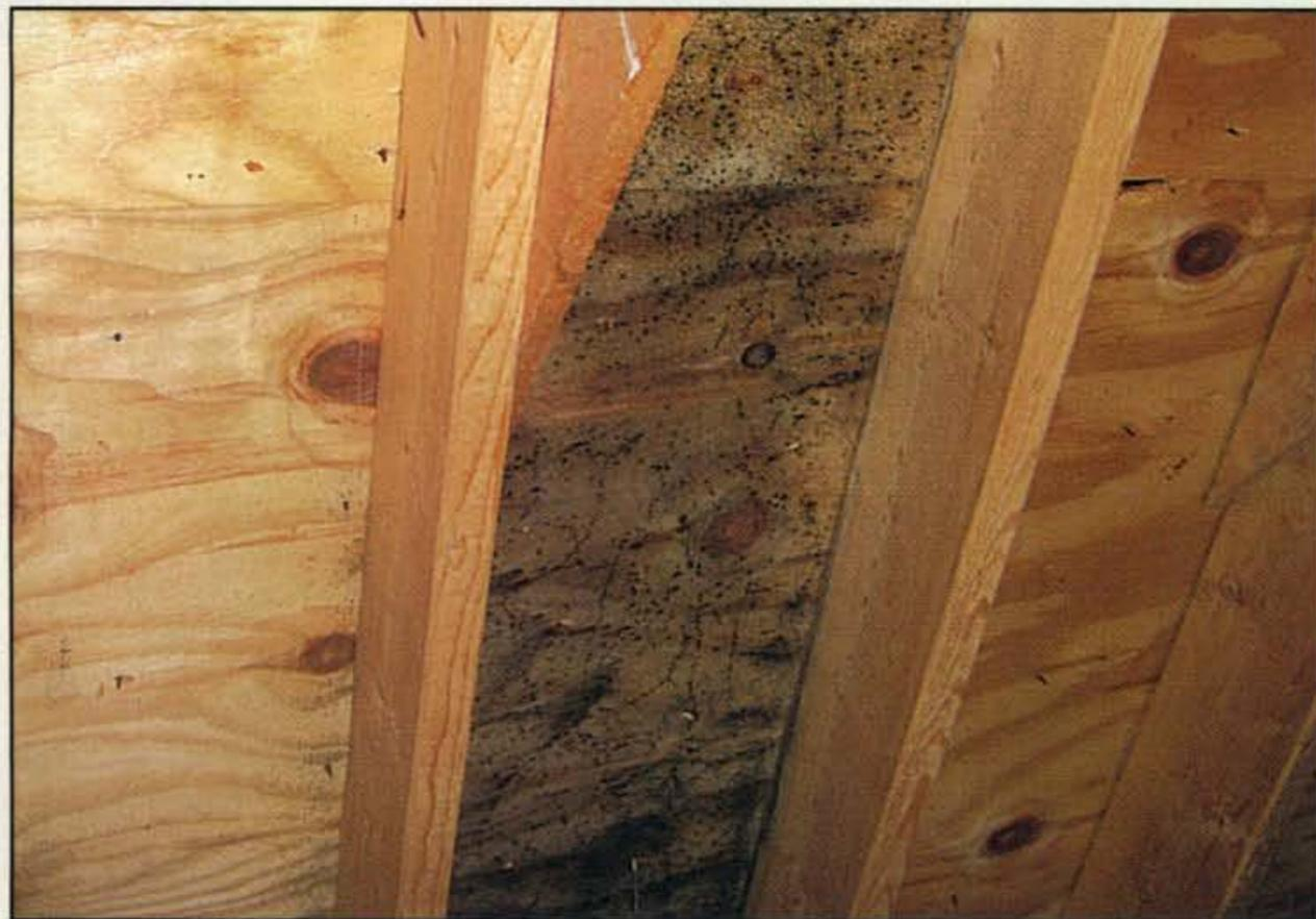
*We were very lucky that this blackened area of our roof, directly below where the lightning struck, was the only visible structural damage from the strike. (Except as noted, photos by the author)*
