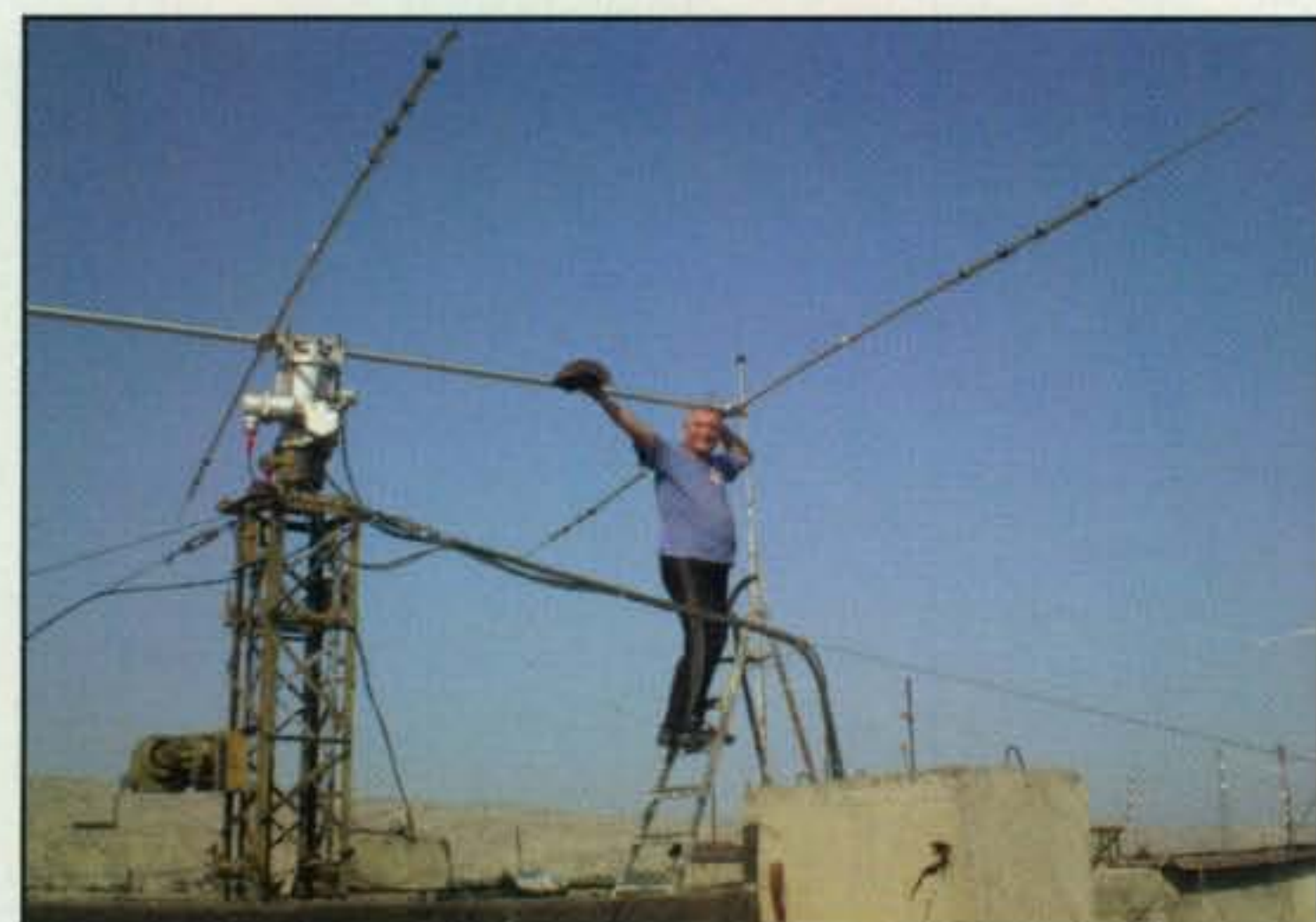
Yuri, 4J3M, doing a bit of maintenance on one of his rooftop antennas. His antenna "farm" is high above the city of Baku on top of the apartment building. (Photo courtesy of DJ9ZB)
