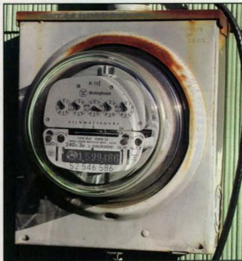
*An old-fashioned “dumb” electric meter that needs to be read manually by a meter reader.*
