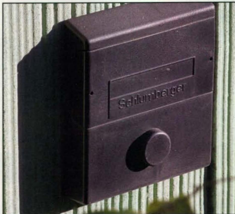
This is an AMR (Automated Meter Reading) transponder for a water meter. It transmits usage data via radio when queried by a meter reader walking or driving past.
