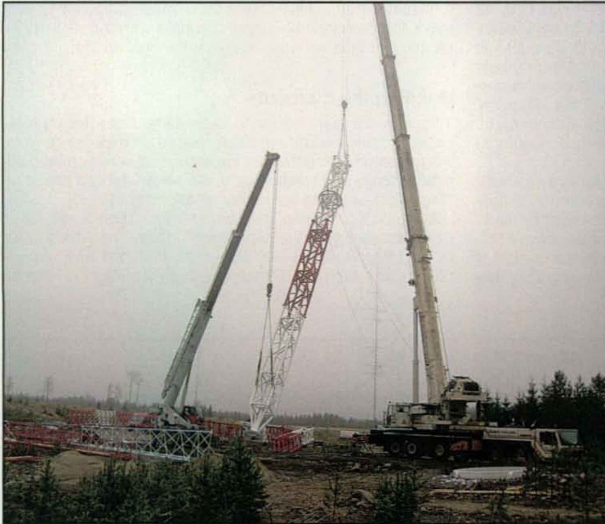
Photo E— Building the tower and antennas took some three weeks, using two cranes. The smaller crane fed the parts to the bigger crane, which then lifted the parts to the men up on the tower, who mounted the pieces together. Photo on left shows the tower base being lifted into place, while photo on right shows upper section being moved into place.
