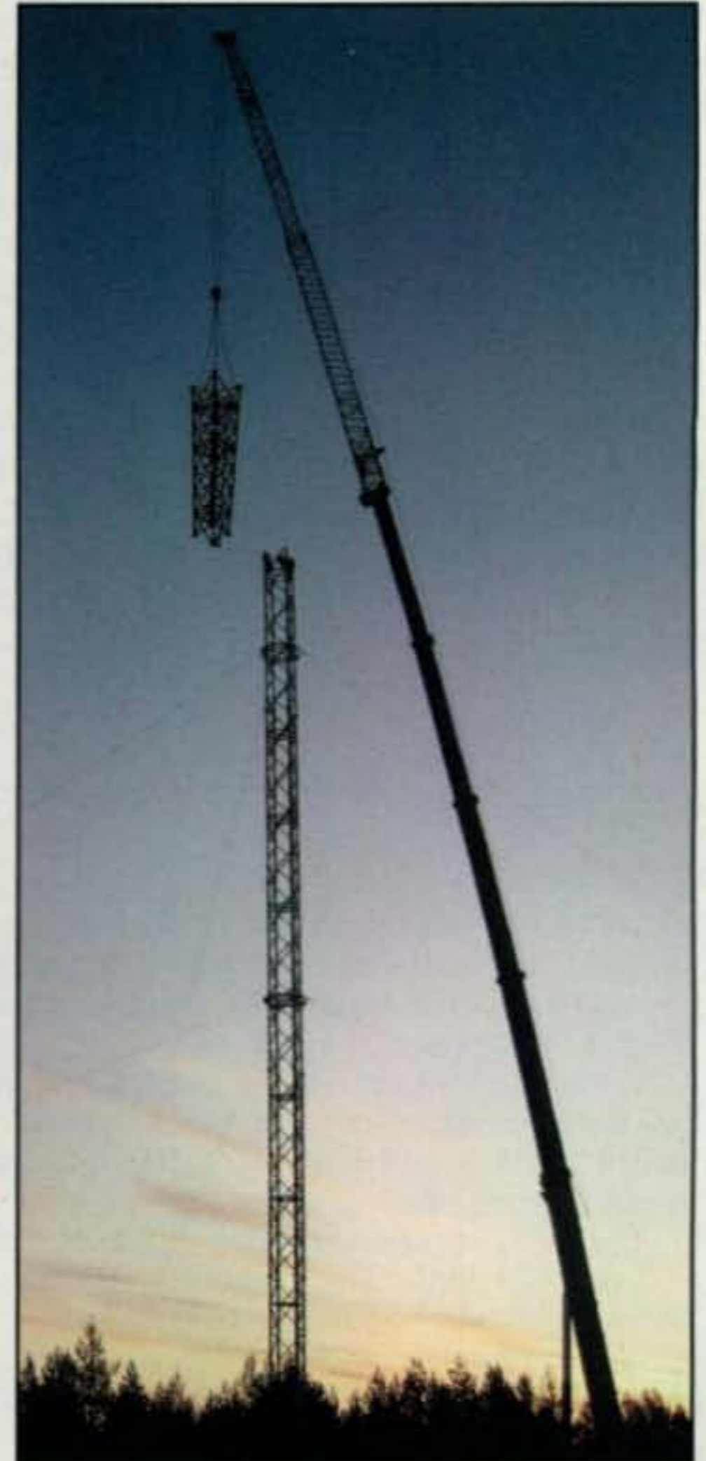
Photo E— Building the tower and antennas took some three weeks, using two cranes. The smaller crane fed the parts to the bigger crane, which then lifted the parts to the men up on the tower, who mounted the pieces together. Photo on left shows the tower base being lifted into place, while photo on right shows upper section being moved into place.
