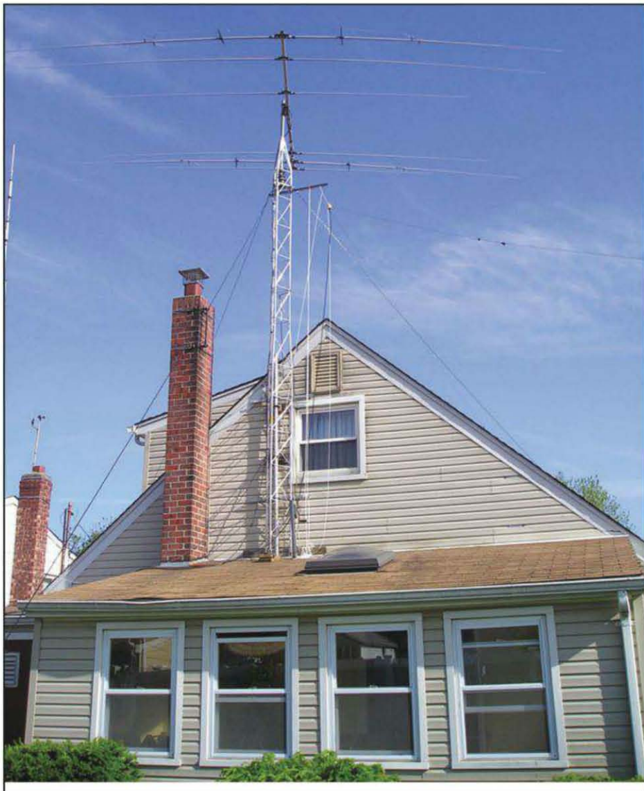
This is Phil's main HF antenna, a Force 12 C3SS Yagi mounted on a small roof tower. An antenna like this is a significant upgrade over a dipole. Upgrading wire antennas to a directional beam will make your signal more readable in contests.
