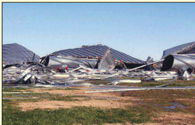
Photo H— An EF2 tornado destroyed grain bins along Arkansas Highway 88 at Sweden in Jefferson County, Arkansas. (Courtesy of NWS)
