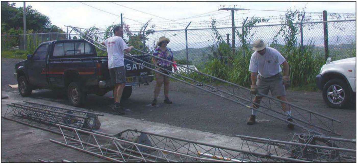
Ulf DL5AXX (left), Diane K2DO (middle), and George N2GA (right), assembling tower sections prior to the contest.
