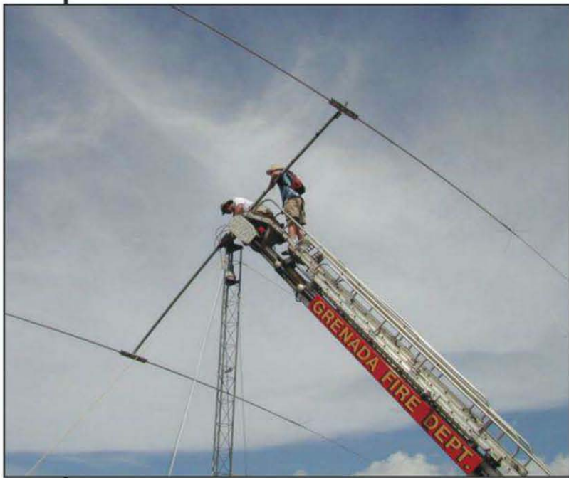
George N2GA, on top of the Grenada Fire Department truck installing a 2-element, 40-meter Yagi as part of the 2006 CQ WW DX SSB Contest DXpedition to Grenada. (All photos by George, N2GA, and Diane, K2DO)
