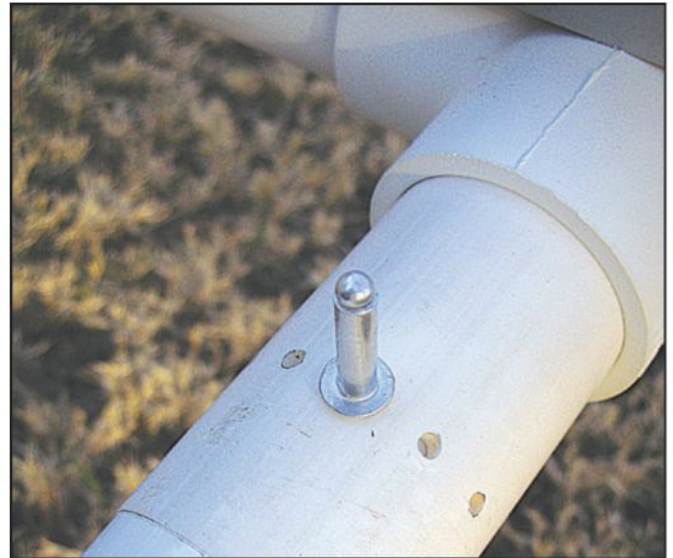
Photo L– The index pin installed to lock the panel in position. Remove this pin to rotate the panel.
