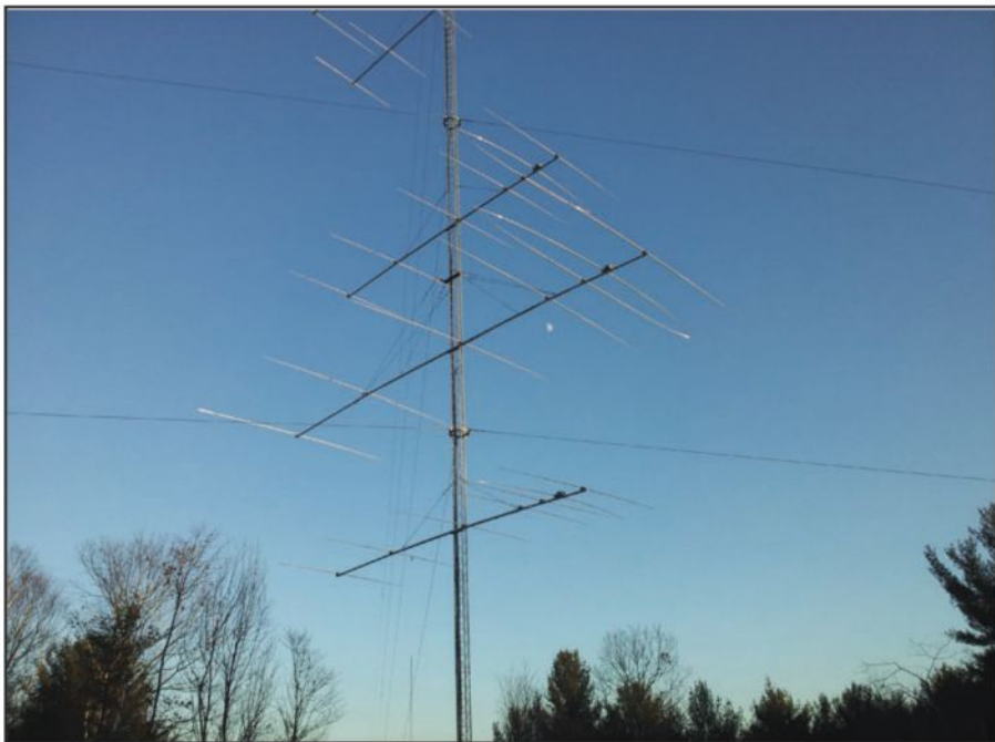
Photo K— Original Tower 3 at WW1WW, showing details of one of the Diamond Drive LFAs on 15 meters and two of the 10-meter OWA Yagis. This tower has now been moved and reconfigured. See text for details. (KØDQ photo)
