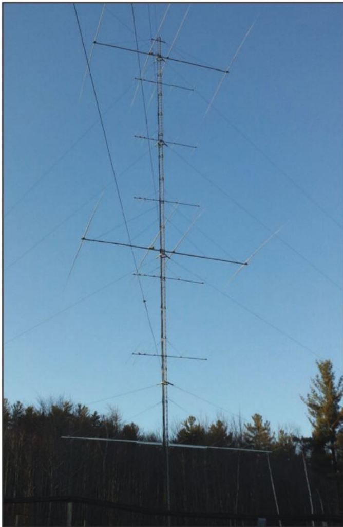
Photo I. Tower #1 at WW1WW: 200-foot rotatable tower with 4-over-4 OWA on 40 meters, six 5-elements + 9-element LFA on 10 meters. (WW1WW photo)
