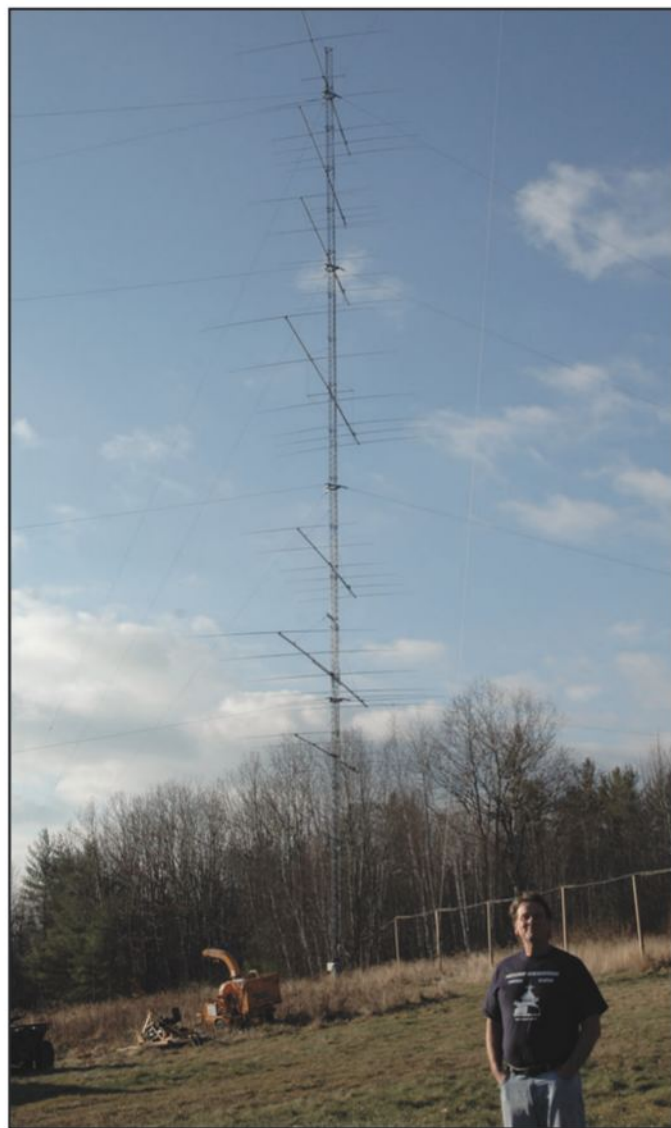
Photo J. Woody, WW1WW, at the base of Tower 2, which holds three stacks of 6-element Yagis on 20 meters and 15 meters, plus a 7-element Yagi on 10 meters. (KØDQ photo)
