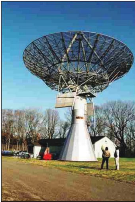
Photo 7— The TLM-18, the 60-foot tracking dish antenna. Photo courtesy ARRL.
