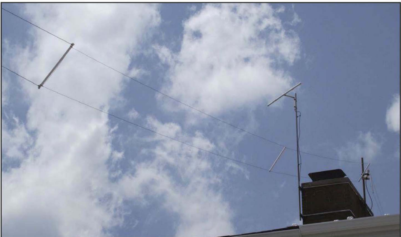
Photo C. One of the ham station antennas at The Seeing Eye.
