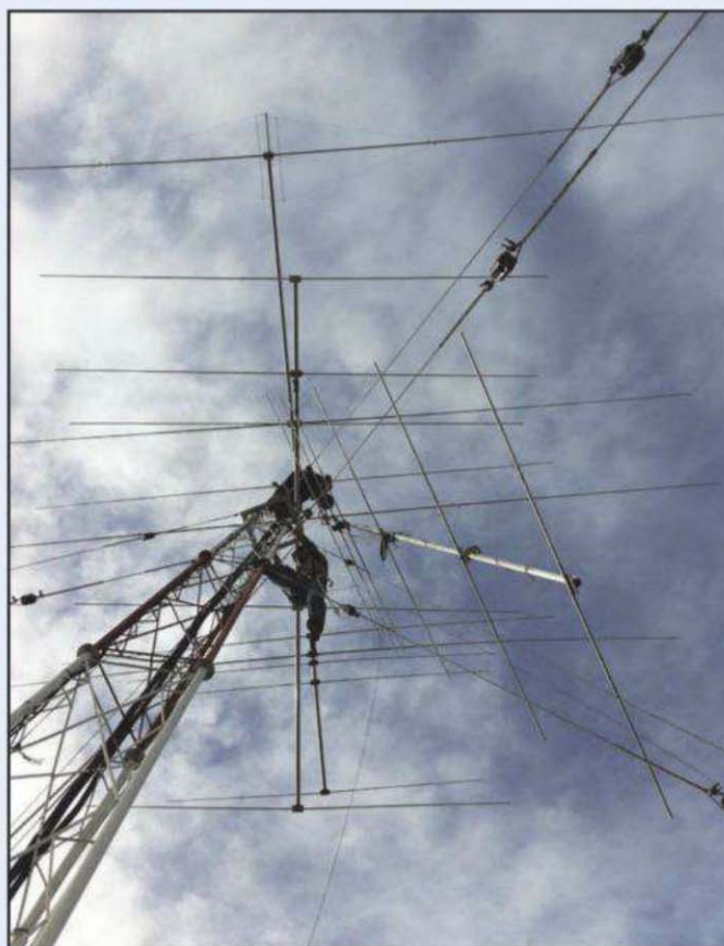
The 6-meter antenna array being set up.
