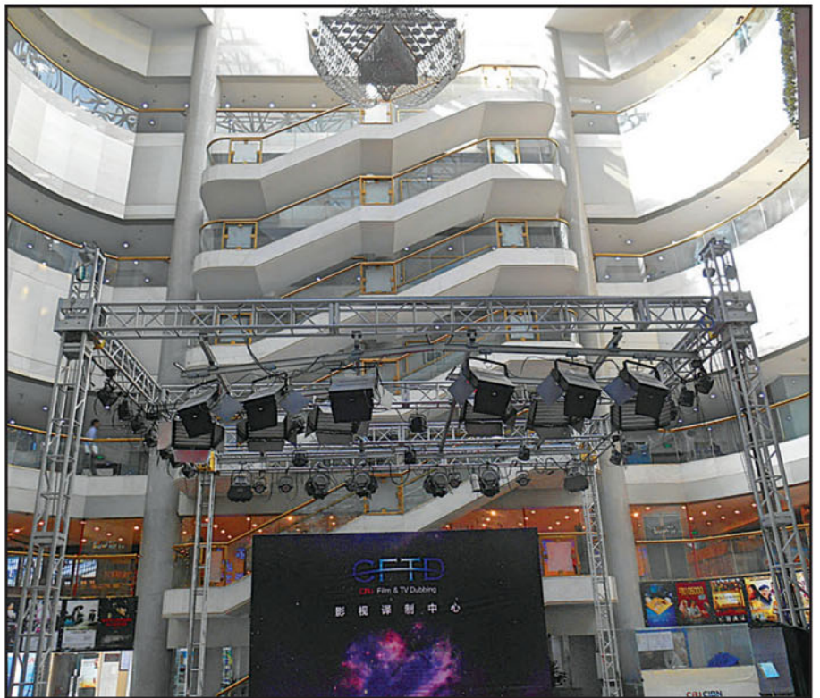
There is nothing understated in the facilities of China Radio International — housed in a 17-story building with a 7-story atrium in a Beijing suburb. (Photography courtesy of KWØU)
