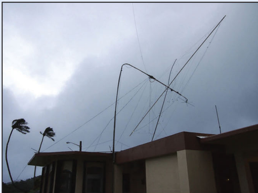
Antenna damage after the tropical storm.
