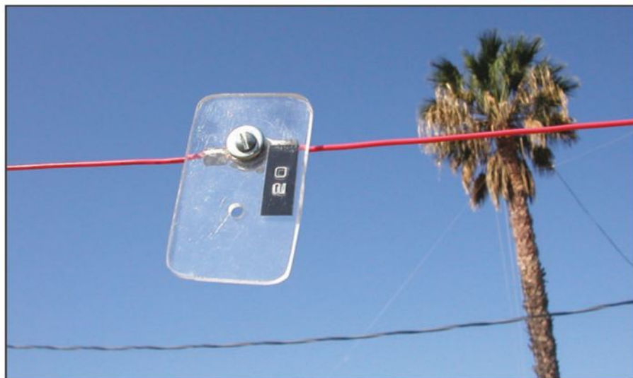
When in "bypass" mode, the solder lugs are connected via the wing nut and bolt, in this case making the 20-meter segment just another part of the longer antenna.
