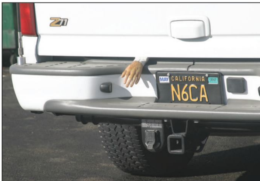
Photo A. The funny fake arm sticking out of N6CA's vehicle inspired a power cable solution for a portable power source from the car battery.
