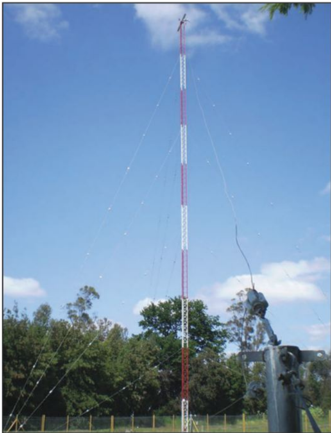
Photo B. Vertical incidence HF radar antenna used for ionospheric research in Chile (Courtesy of CE5BQD)
