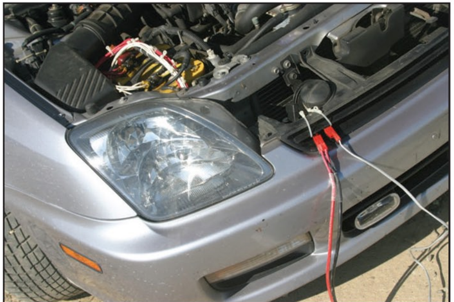
Photo C. Here is a safer, cleaner way to access power from the car battery. Multiple wires are routed from the battery terminals and under the car. The gray wire on the right is a small-gauge pair of wires going to a set of solar panels.
