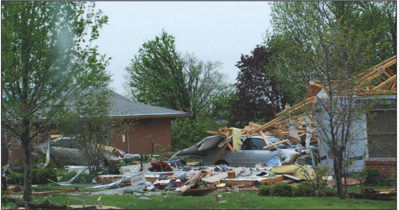
Photo G: Good Friday, April 23, 2011 EF4 tornado storm damage in St. Louis.
