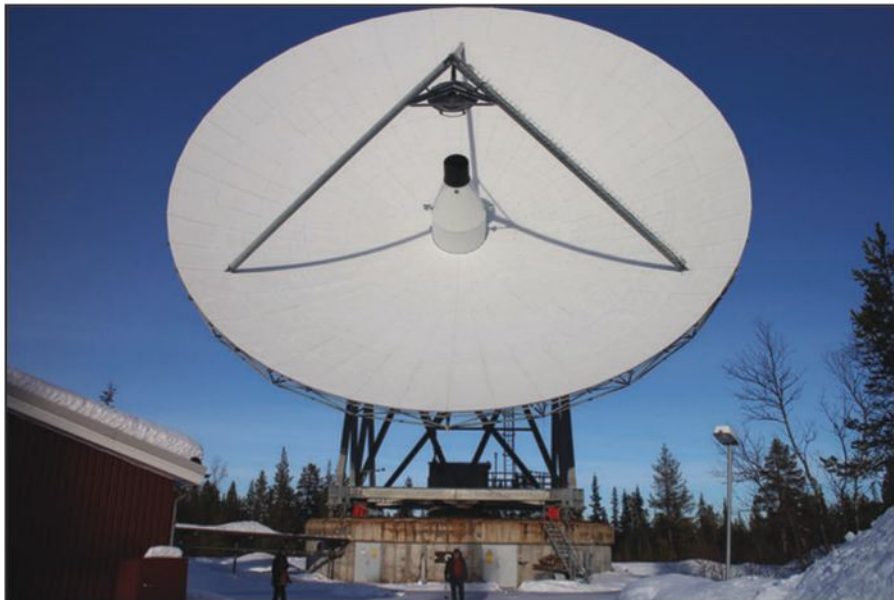
Photo A. The 32-meter parabolic dish antenna at Kiruna, Sweden. This is part of the EISCAT research facility and not used for ham radio (Photo courtesy Dr. Craig Heinselmann)
