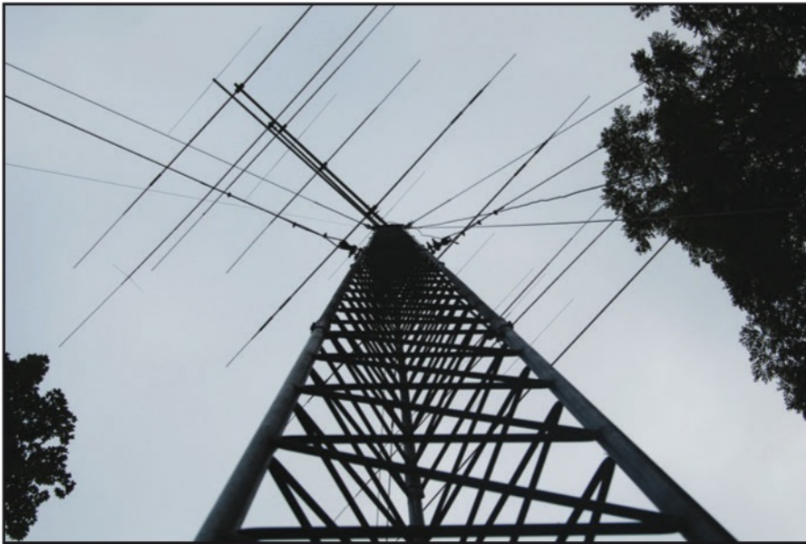
Photo C. Looking up the tower at the RemoteHamRadio location in Quaker Hill, New York ... something apartment — or HOA — bound hams used to only be able to dream of using. (Photo by Lee Imber, WW2DX; courtesy RemoteHamRadio)
