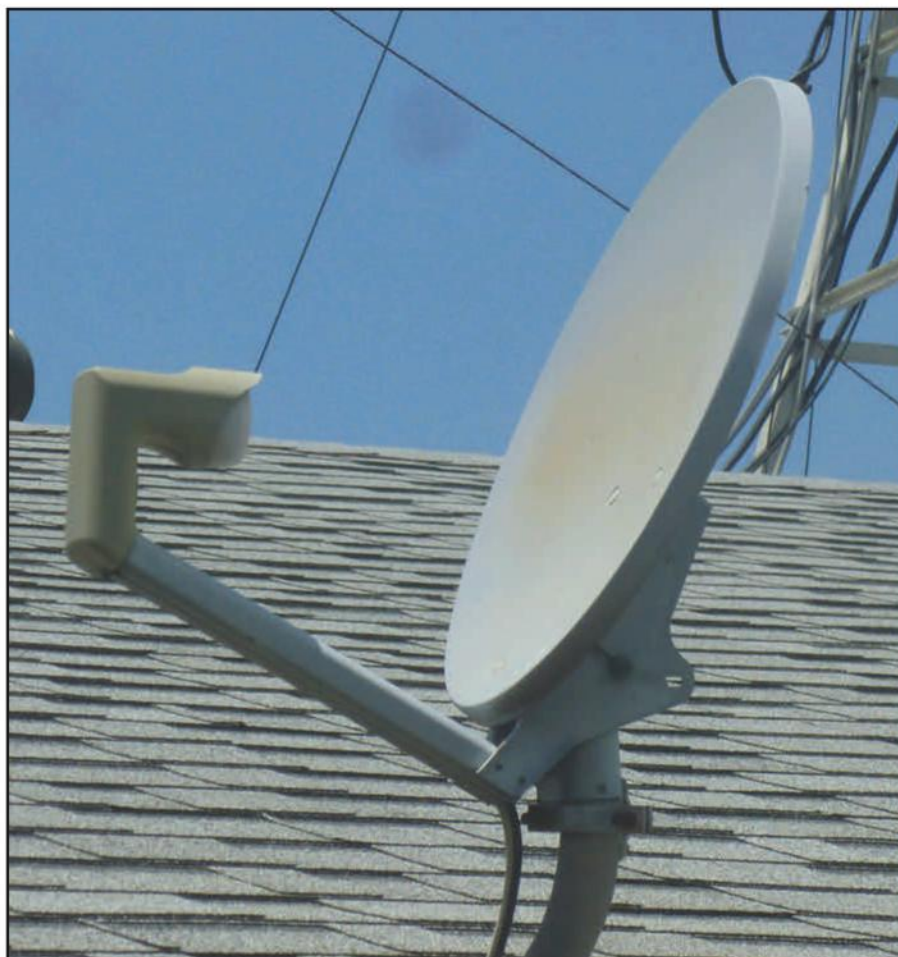
Photo A. Offset feed satellite dish.
