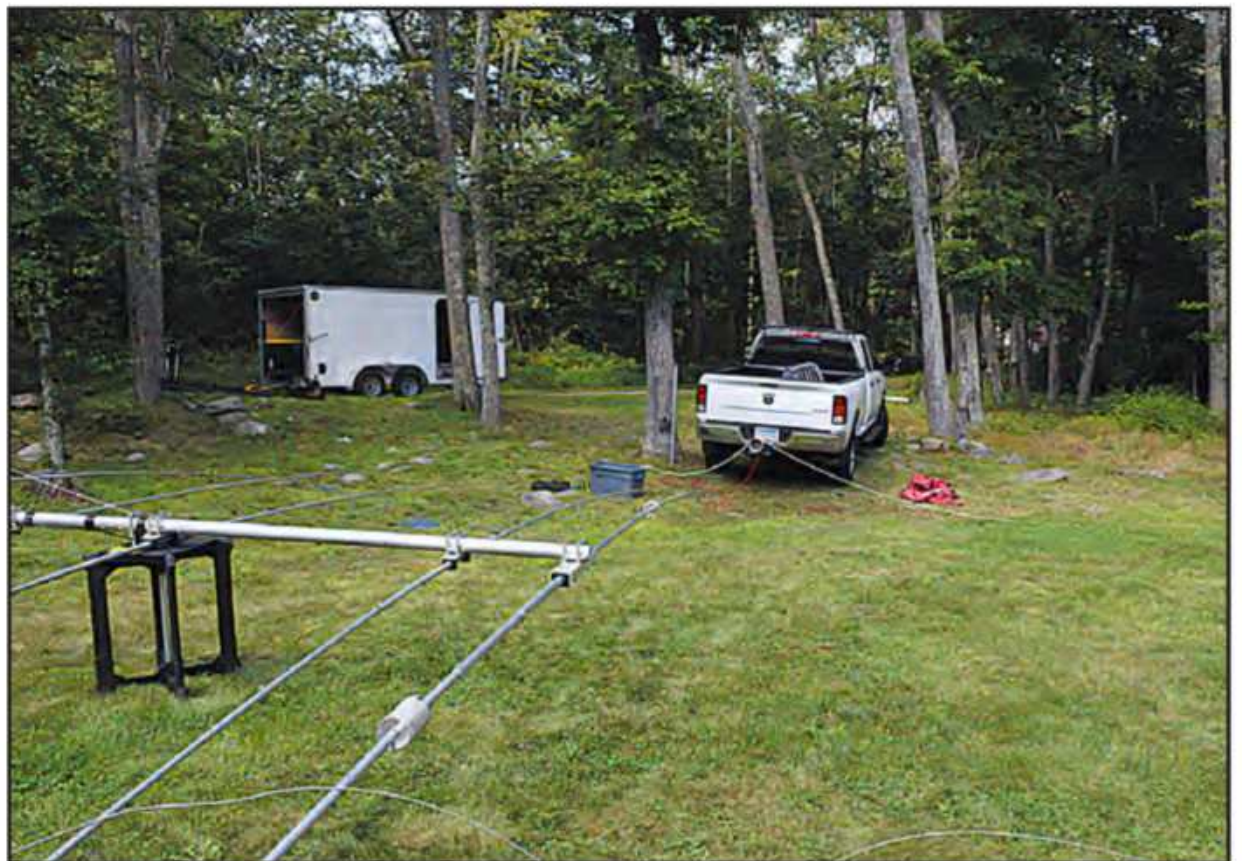
Photo D. Antenna removed from tower, prepared for disassembly, and removal by HamEstate.
