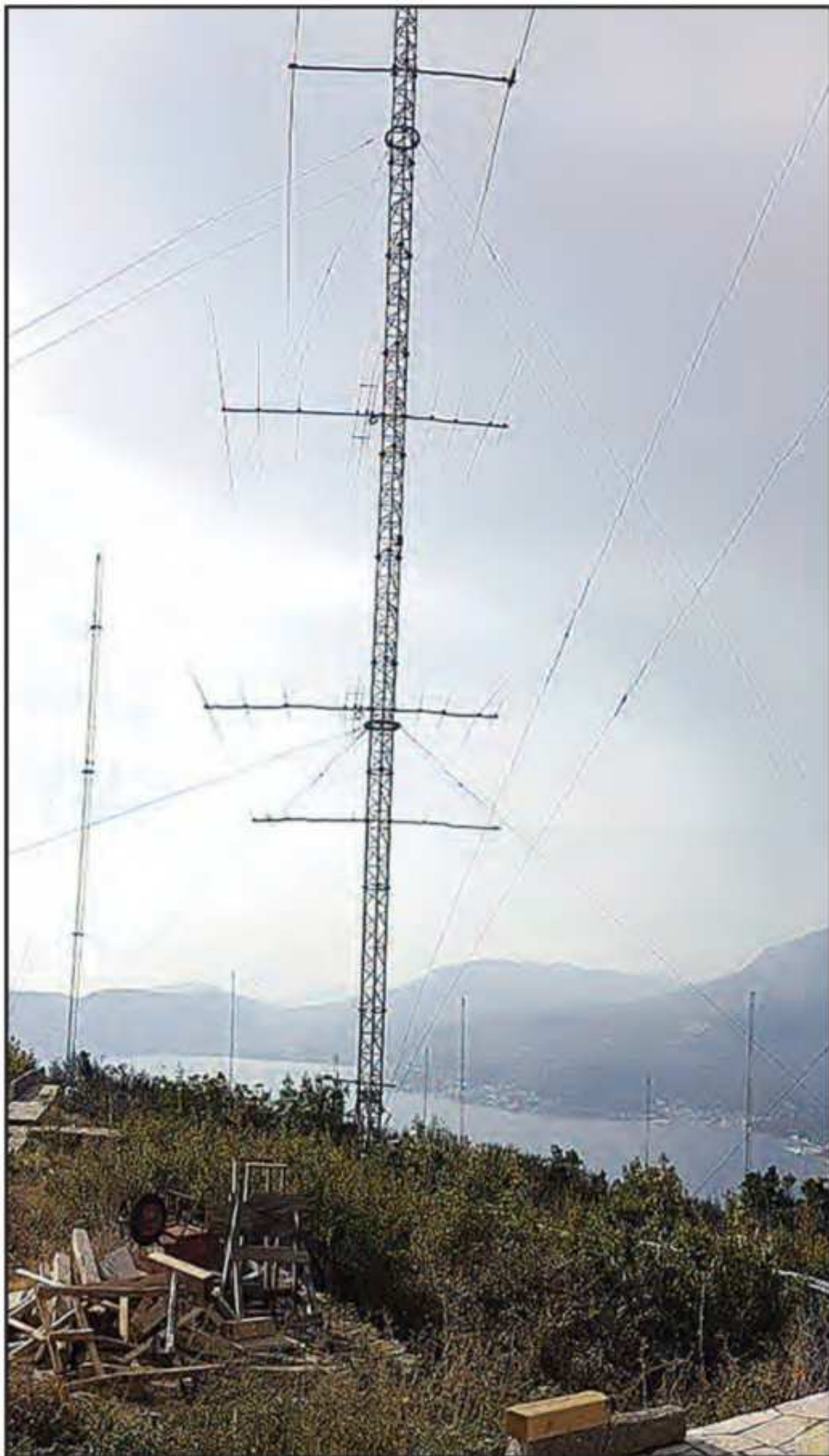
The beginning of 4O3A's new towers and antennas overlooking Kotorška Bay in Obosnik, Montenegro. Pictured is the first tower and multiple antennas completed in August 2018 for use by the Region 1 IARU Youth Team in September's CQWW RTTY contest. From top-to-bottom: 2 elements for 40 meters, 2 X 10/15/20 meter multiband stack, and 6-element 6-meter Yagi. (Courtesy of 4O3A)
