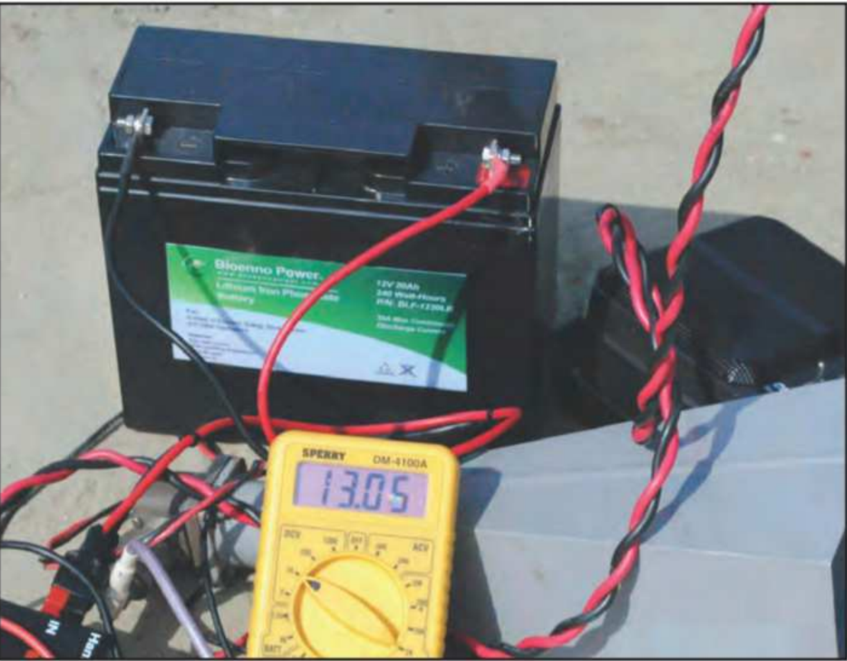
Photo F. Bioenno battery that ran all through Field Day, still ready to work.
