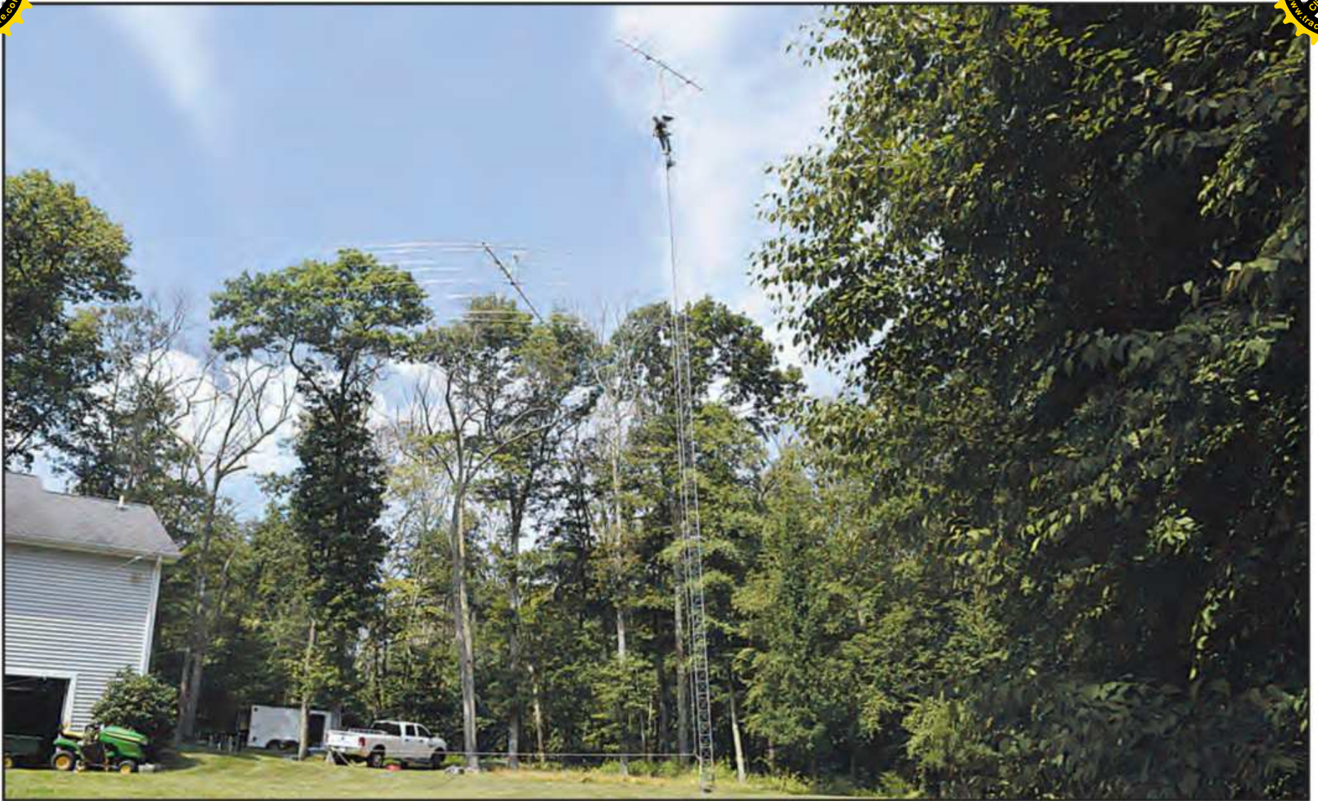
Photo C. HamEstate crew member trimming down a 240 pound HF yagi antenna for disassembly. (Photos C, D, E courtesy of HamEstate)
