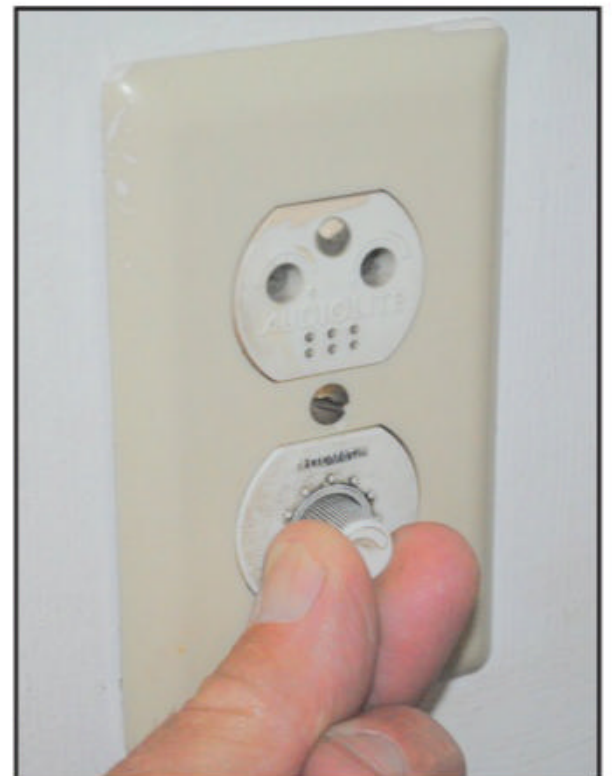
Photo B. Dimmer circuits create major static on HF band reception.
