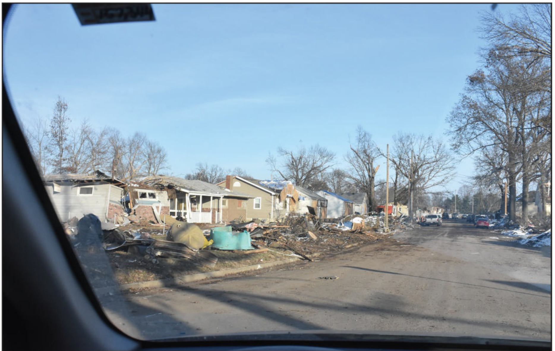
Photo A. Extensive damage along a Taylorville, Illinois, street from a December 1, 2019 EF3 tornado. (Photos by the author, except as noted)
