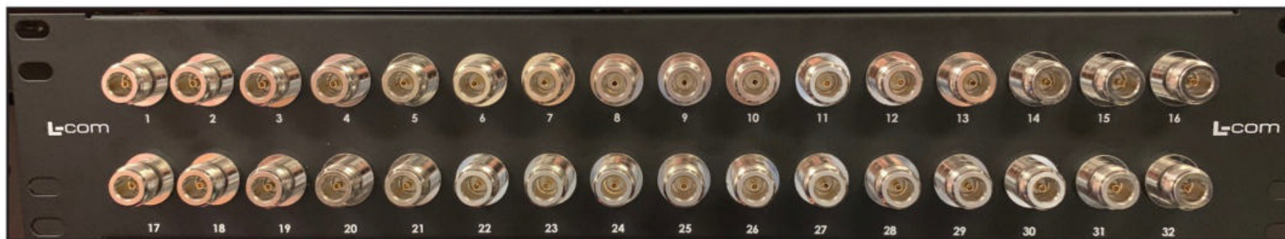
Photo O. Antenna patch panel 3.5-inch (2U), 32 N-type 50-ohm connectors (L-Com Item # PR35N32BLK or PR35N32CMB). Cables from antennas enter back of patch panel (top row); cables to radio transceivers exit back of patch panel (bottom row).
