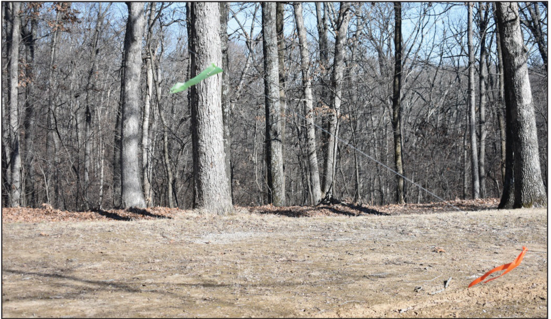
Photo F. Note the safety “flags” placed along guy wires to make them more visible to passersby.
