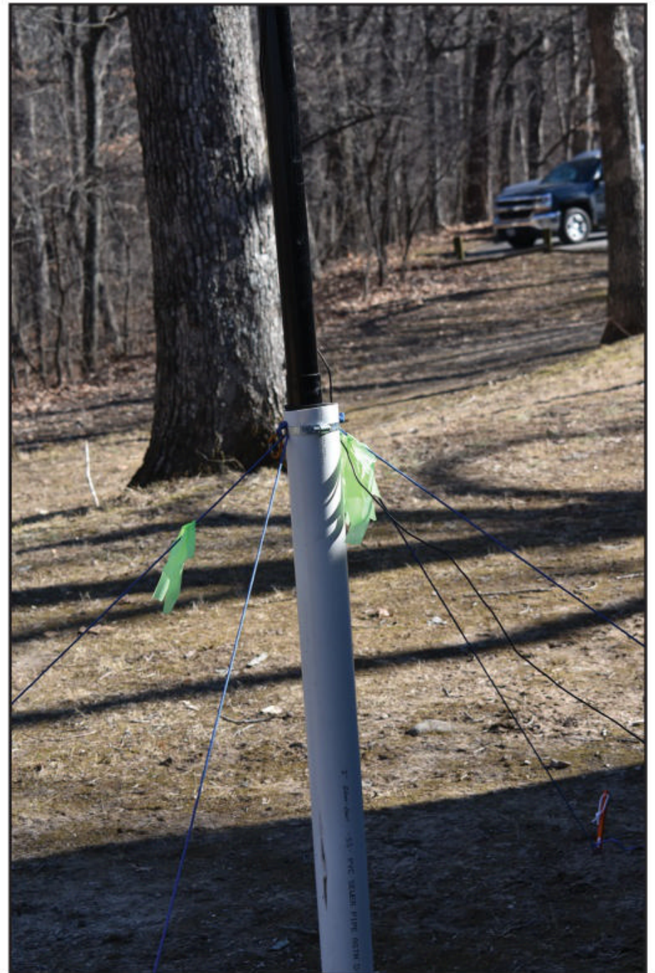
Photo E. Ground radials from the Aerial 51 off-center-fed dipole (OFCD) used by SLQS.
