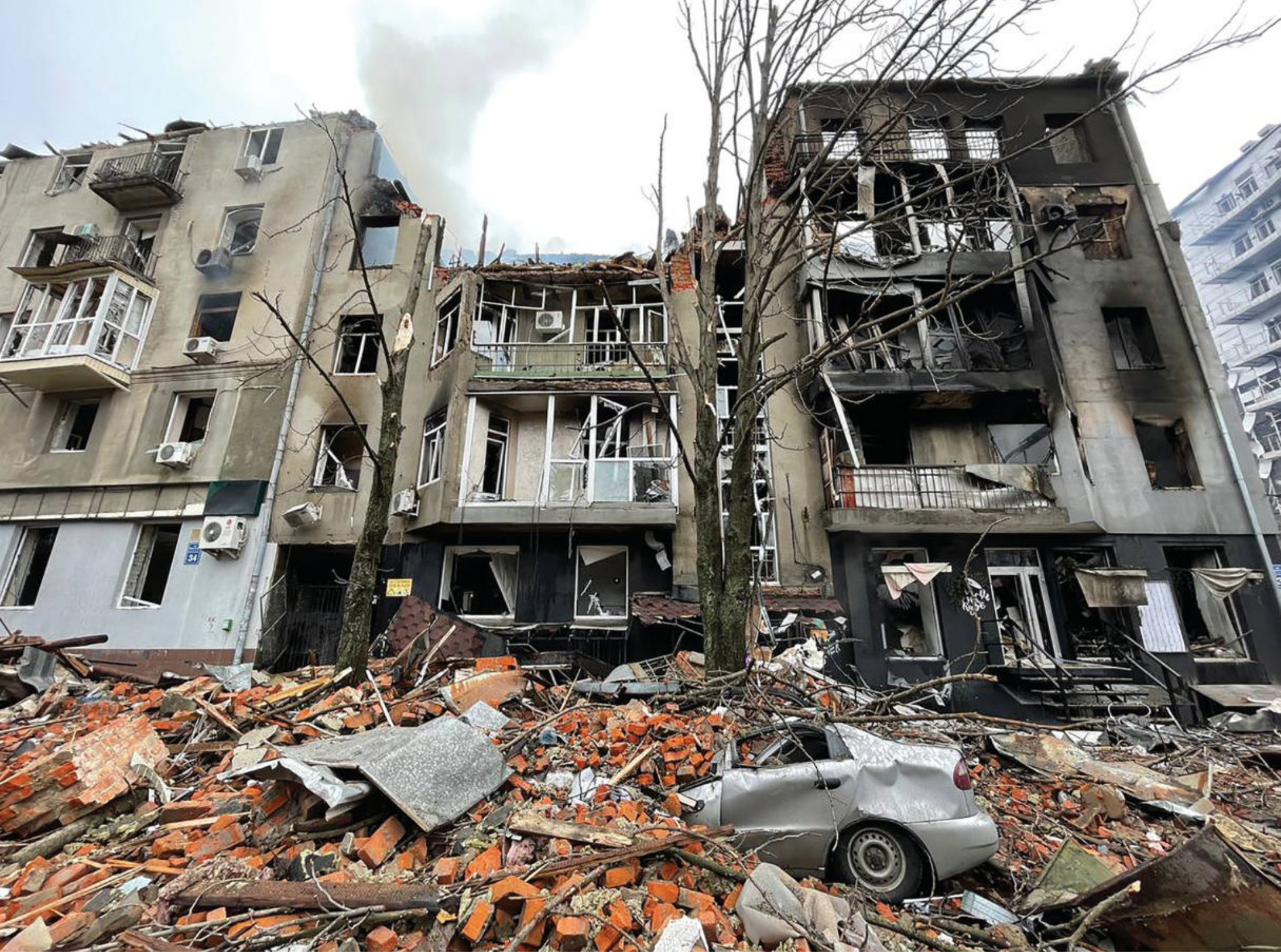
Bombed-out apartment building in Kharkiv, Ukraine. (Photo courtesy Depositphotos.com)
