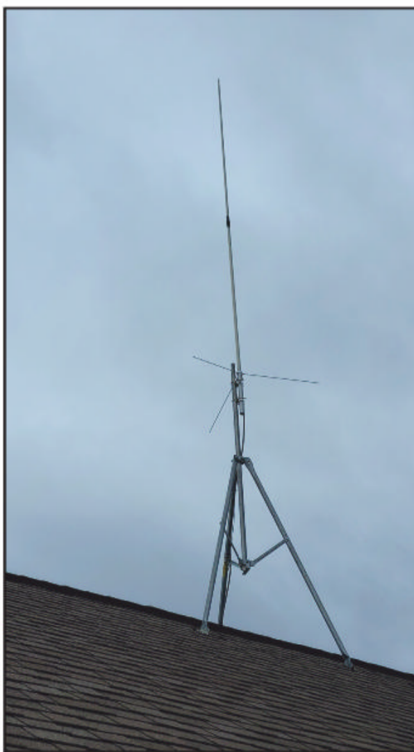
Photo B. NØBMK's roof-mounted dual-band antenna. (Photo by Brian Koch, NØBMK)
