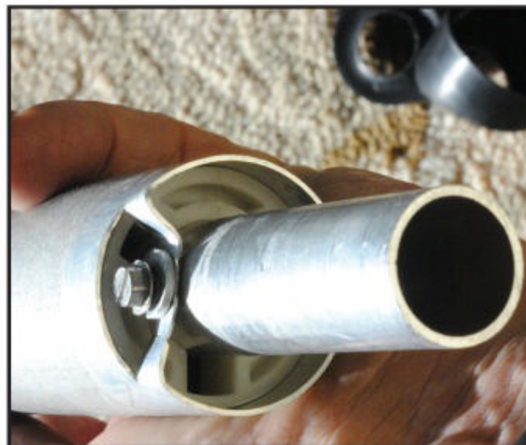
Photo I. This self-tapping screw underneath a trap’s bug cover may need to be tightened.
