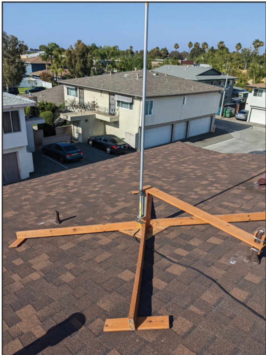
Photo C. The vent-pipe anchor also helps keep the antenna vertical on a sloped roof.
