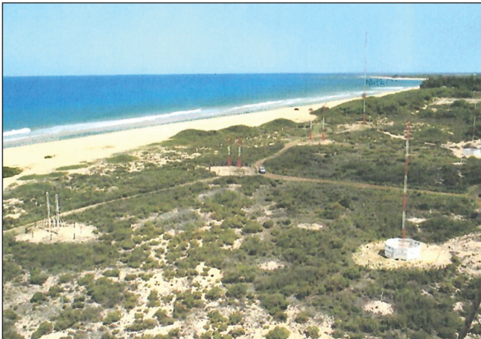
The antenna field at WWVH, Hawaii, WWV's sister station in the Pacific.
