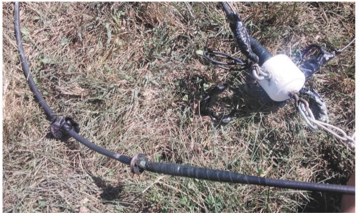
This image shows the offending stand-off insulator where high voltage from the coax shield arced across the plastic spacer to the metal eyelet and on to ground. The excess tape that trapped moisture can be seen above and below the eyelet. (Courtesy of W3TS)
