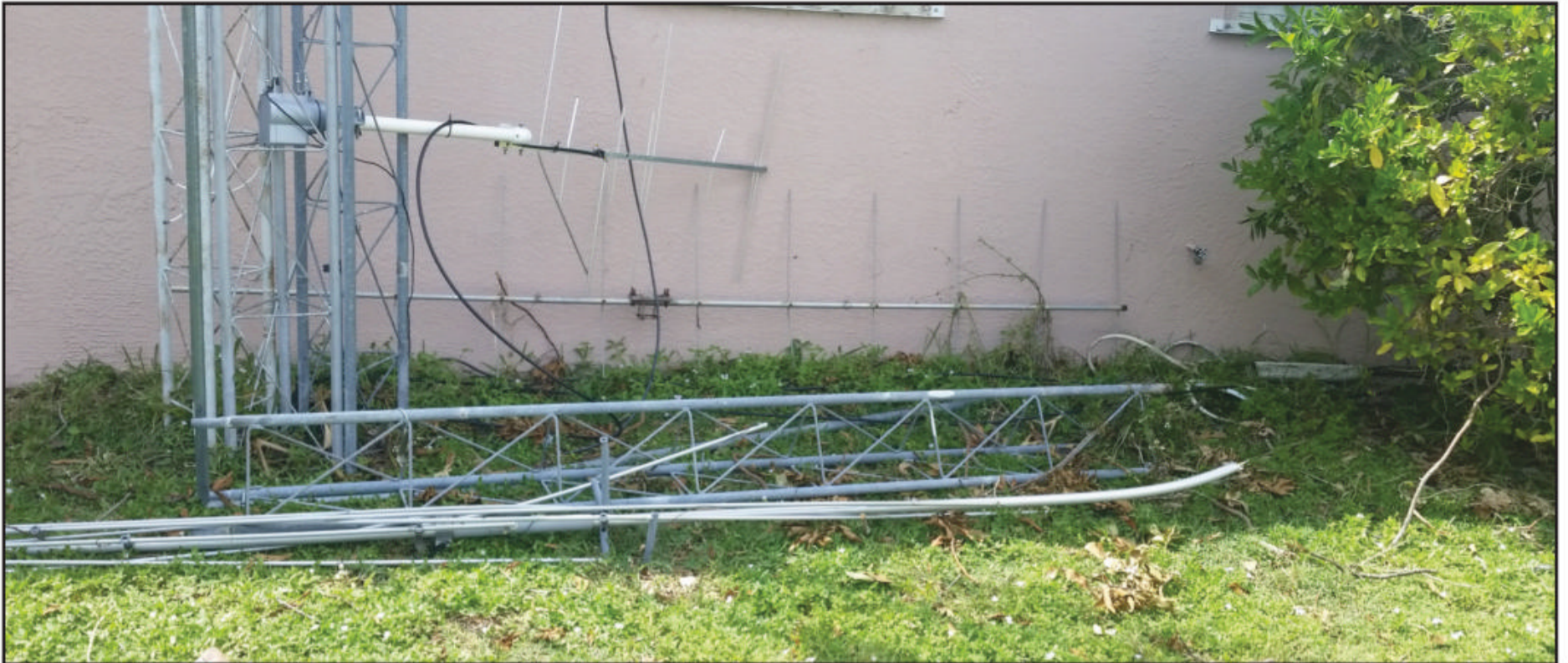
Photo B. I think the rotor survived but my beams are missing multiple elements.
