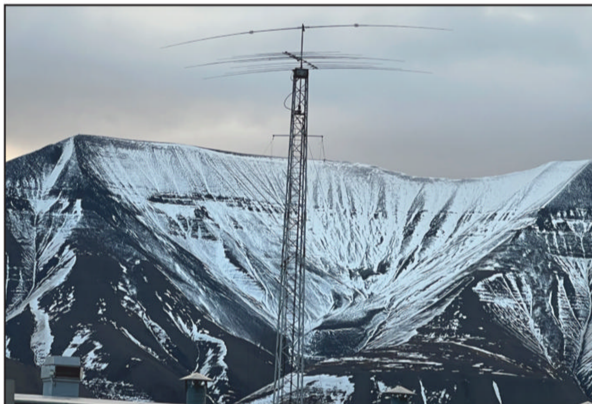
Photo C. The main tower at JW5E is 26 meters/85 feet high. See text for antenna details.
