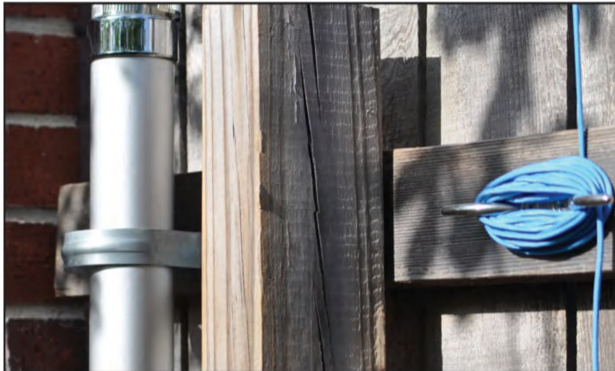
Photo D. The pole is clamped to the fence where the cleat is installed.
