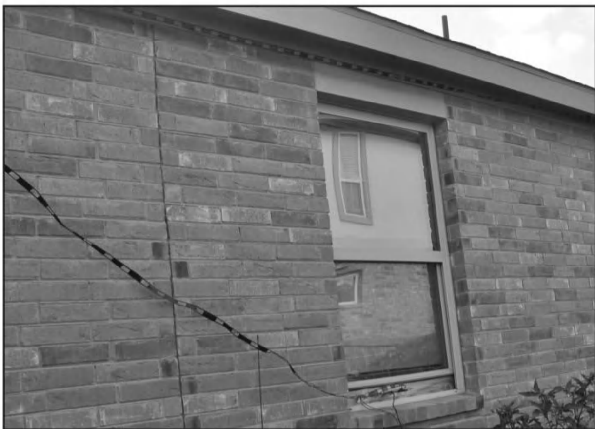
Photo A. The ladder line runs under the lip of the roof for most of its length.
