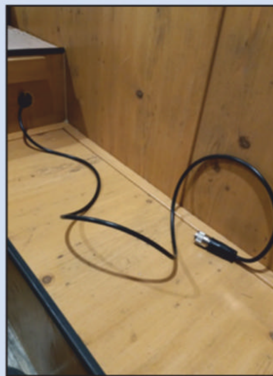
Thru Holes drilled through seat and wall. Cable reaches radio on table.
