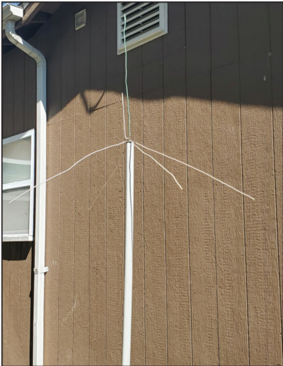
Photo A. Back on the air again ... wire ground plane on PVC conduit
