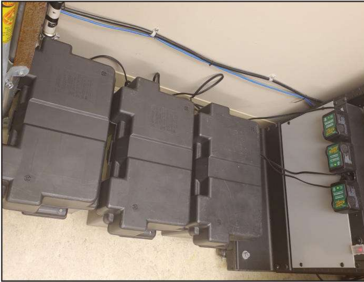
Photo D: Three 100-amp/hour Group 27 AGM batteries for the “go kits” in battery boxes. All your standby batteries for your home station should be in boxes like these for safety.
