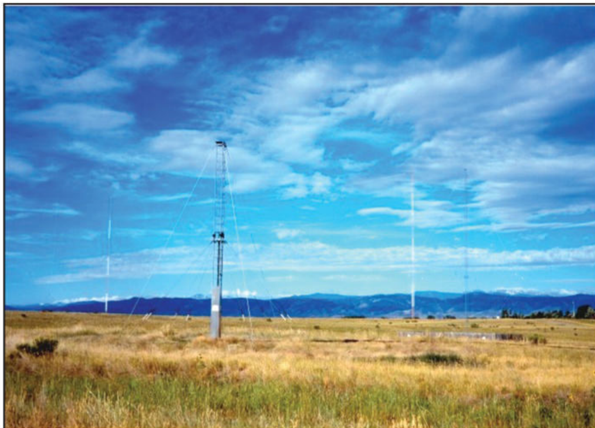
Photo F: One of radio station WWV's omnidirectional HF antennas near Ft. Collins, Colorado.
