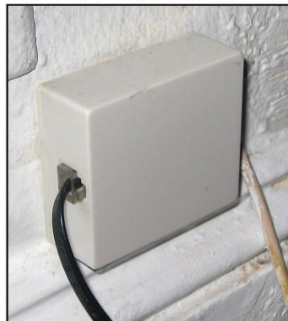
Photo B: A household telephone jack for a phone line’s twisted pair of wires. (Photos B-F from Wikimedia Commons)
