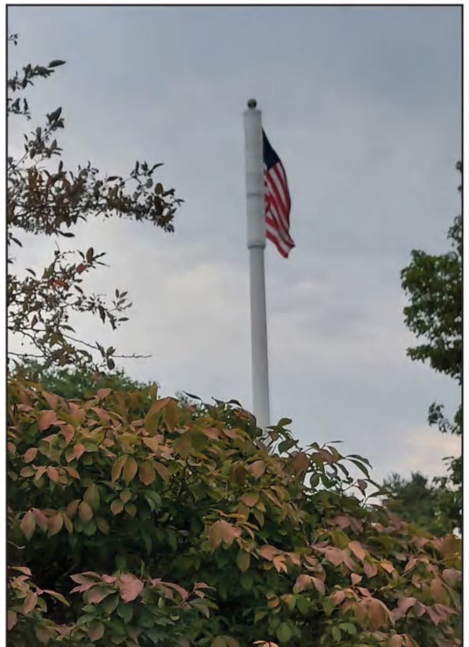
Photo A: A suburban cell phone tower masquerading as a flagpole in an area with antenna zoning restrictions.
