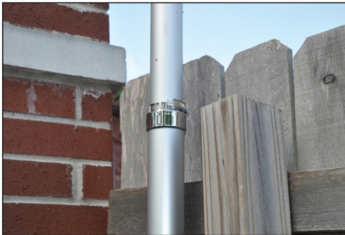
Photo C. Pipe clamps prevent each telescoping section from collapsing.
