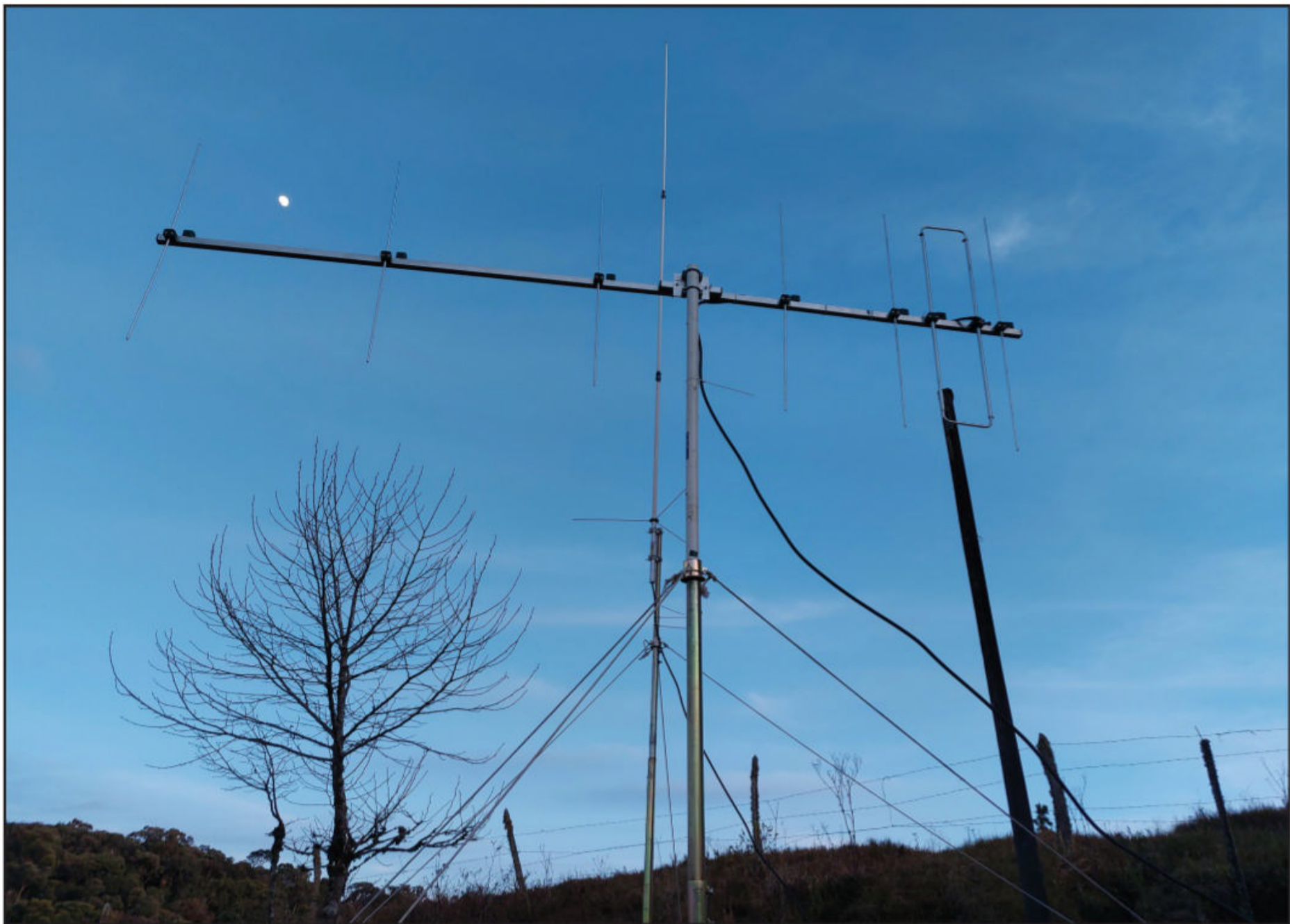
PY2QB's antenna farm — a 7-element LFA Yagi and an omni vertical. (Credit: Ricardo Benedito, PY2QB)
