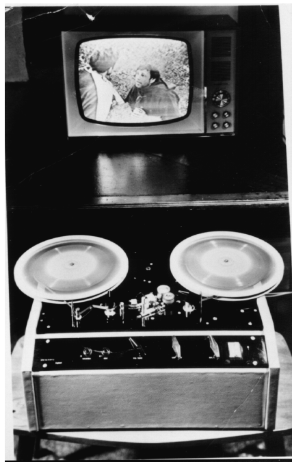
Telcan unit playback demonstration at its launch in 1963. The early prototype (1962) model is shown in the heading.
