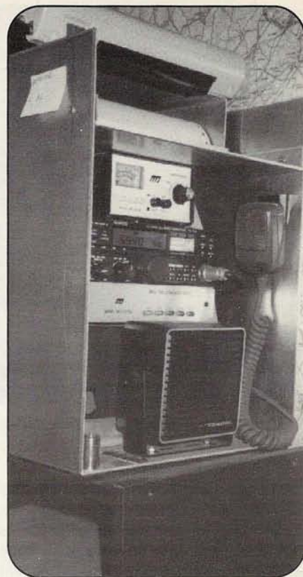
The portable set-up used for the TRIAGE database: Diconix printer on top, 12 volt MFJ power supply sitting on Kenwood TR-751A, on top of MFJ 1270B. Base holding aluminum stand fits over "hump" in vehicle.
