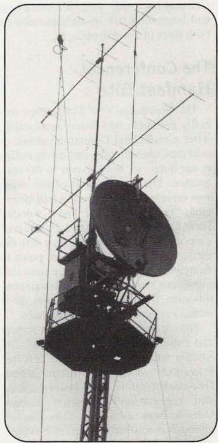
Photo E. One of the VHF/UHF towers at the Weinheim club station. The towers were surplus from electrification of Germany's light rail system.
