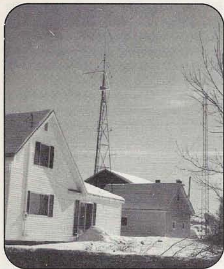
Antennas and towers didn't fare much better than trees in the northeast ice storm, meaning that public service agencies tied to permanent antenna installations were also cut off, increasing reliance on hams and their flexibility in setting up temporary stations. (WX2DEB photo)
