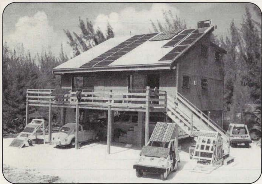
Photo B. Solar energy supreme! Panels on roof (approximately 34 of them) mated with a bank of 20 or 30 batteries that are discharged only 10 to 15 percent by daily loads can serve as a quite effective stand-alone power system for home and rig(s). (Photo courtesy Alternative Energy Engineering)
