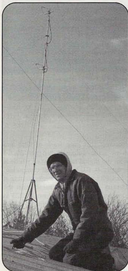
Photo F. NØLL installs a guy wire for the 2-meter Par Triangle antennas. His 2-meter beacon went on the air in February, 1998. The 6-meter beacon's been on the air nearly continuously since 1985.
