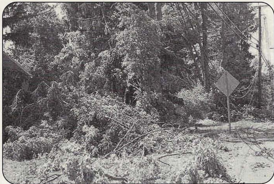
Even where trees were left standing, downed limbs and branches pulled down power and telephone lines, giving hams plenty of opportunity to provide emergency communications in the wake of the storms.
