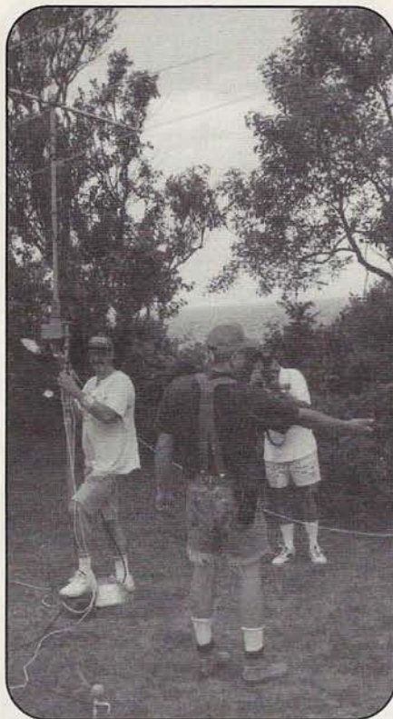
A three-element beam is all that was needed at W2AMC to make 270 contacts on 6 meters during FD. In this photo taken at set-up time, the author is holding the base of the monopole used to support the antenna while club FD Coordinator Don Fisher, N2QHV, and club member Warren Melhado, KG2BI, prepare to guy the "tower." Fully extended, the monopole put the Yagi 20 feet in the air.
