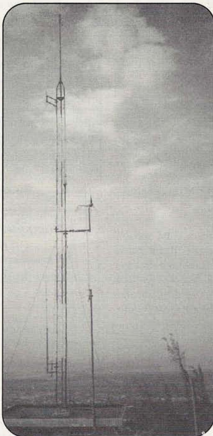
Photo A. The tower, antennas, and wind-powered generator at the Cadena el Conquistador repeater site in Rio Grande, Puerto Rico, about 20 miles west of San Juan.
