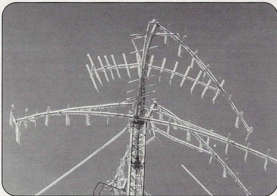
Can you protect your antennas from winter's ravages? WB2D's tips this month will help prevent damage from typical winter weather. On the other hand, a major ice storm, such as the one that hit the northeast last January, will defeat even the best-maintained antenna system, which this was. (Photo courtesy Dave Olean, KIWHS/ARRL)
