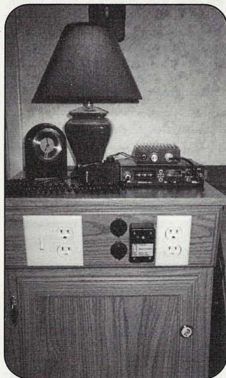
Photo A. Completed emergency-power cabinet posing as a nightstand. The two 110-volt AC outlets connect to DC-to-AC power inverters inside the stand. The two cigarette-lighter plugs connect directly to the 12-volt gel-cell battery inside. (Photos by the author)
