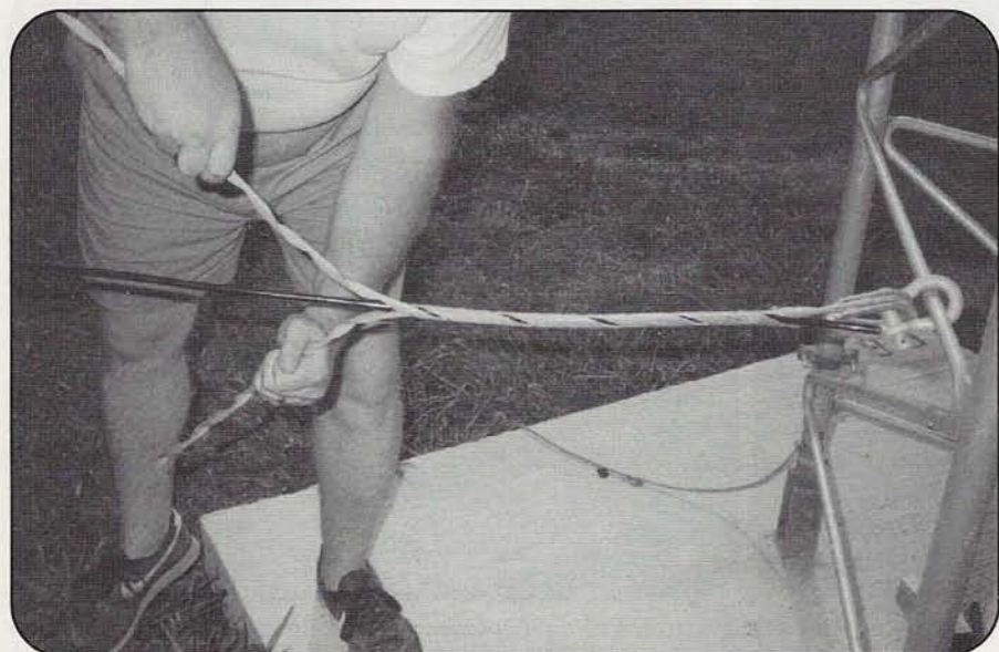
Photo D. Continuing to wrap the Phillystran in the "big grip." Patience will be required.
