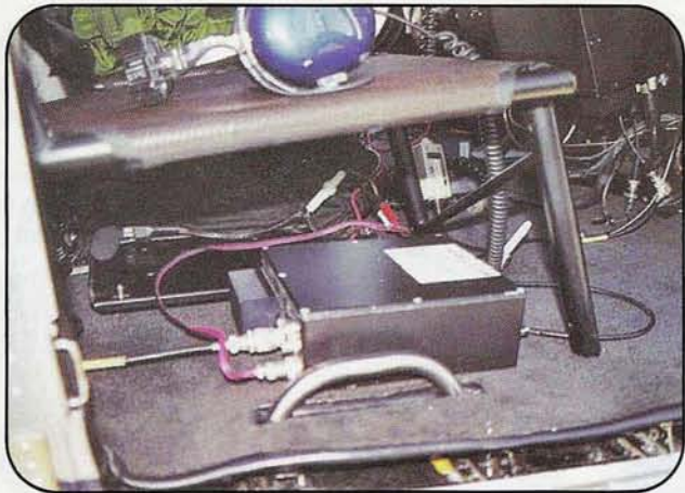
This is the P.C. Electronics 10-watt ATV transmitter inside the helicopter.
