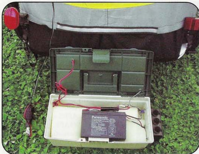
The battery that powers it all. A view inside with the Panasonic 7.5 SLA battery charged via solar power. Notice the three cigarette receptacles for power distribution.
