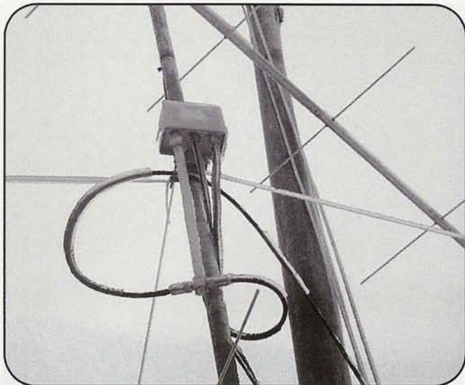
As if their troubles had been few, the VO1AA team arrived at Cabot Tower on the windy third day of the experiment to find antennas and feedlines coated with ice.
