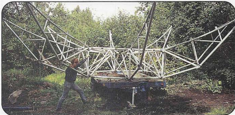
Photo 2. Assembling the support for the dish.
