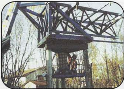
Photo 8. Preparing the base for the dish.
