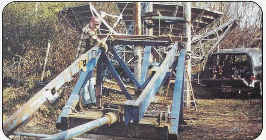
Photo 6. Welding back together the 2 × 6 beams.
