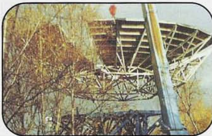
Photo 9. Lowering the dish onto the base.
