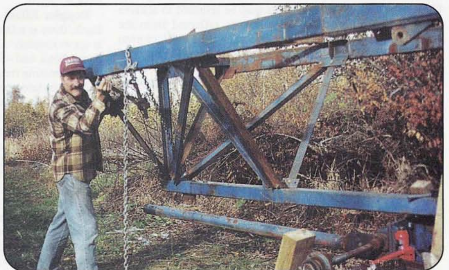
Photo 7. Another view of the professional welder working on the 2 × 6 beams.
