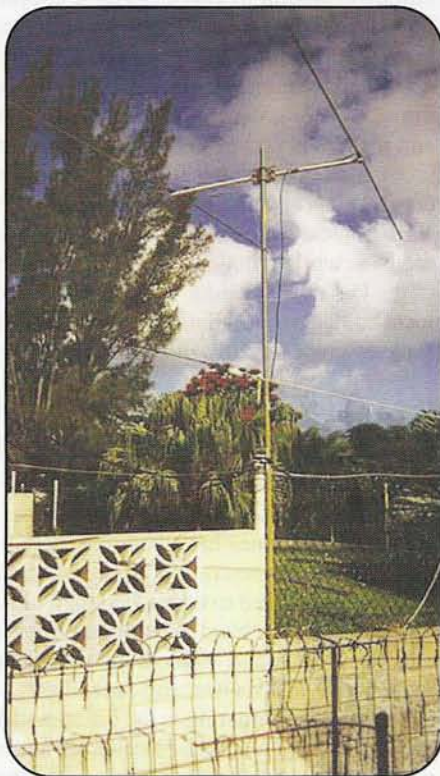
Jon Jones, NØJK, used this simple two-element Yagi with good success during one of his earliest trips to Bermuda. (Photo by NØJK)
