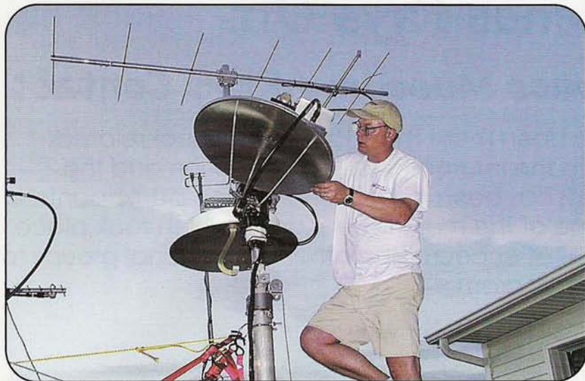
Photo B. KMØT helped NØDQS/R with the final installation of the microwave dishes prior to the 2002 UHF Contest.
