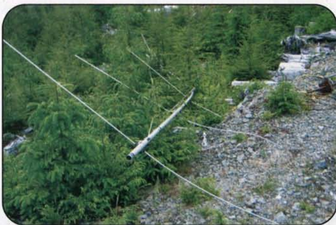
This is what sometimes happens when you have only two people to take down a tower with rotator, mast, antennas, and cables still attached!
