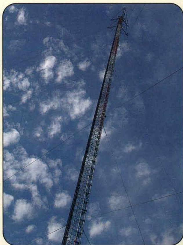
The FRRL D-STAR tower. The FRRL D-STAR systems installation used 1200 feet of 1 5 / 8 Andrews heliac. This required 450 stainless-steel line hangars (at $1.90 each) and 56 man-hours of professional tower-climbing time to complete. (Photo courtesy of Greg, N9CHA)
