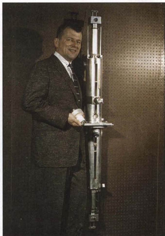
Figure 12. Photo of W2CXY with the "stovepipe final" VHF amplifier, circa 1956.
