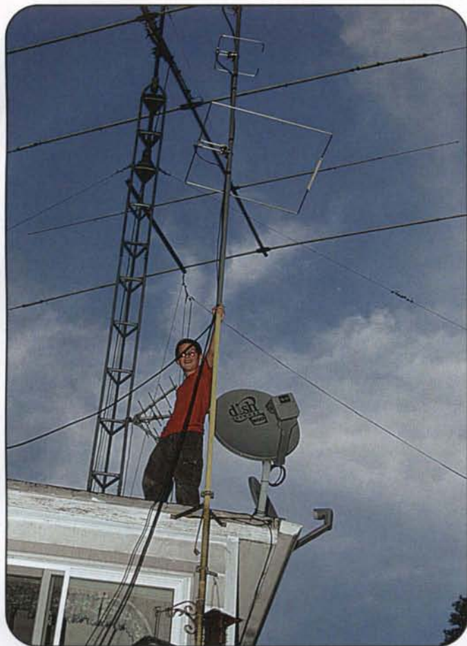
Llyam on the roof holding on to the mast that supports the loop antennas.
