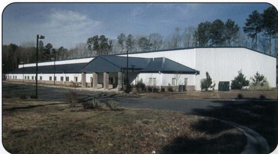
The new AMSAT Laboratory in Pocomoke City, Maryland. (AMSAT photo)
