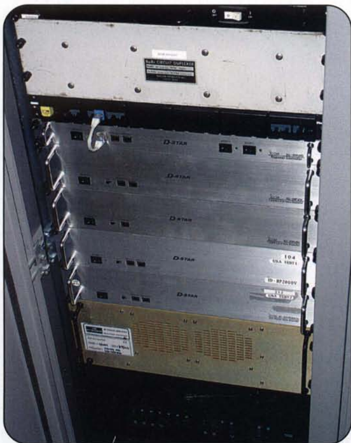
The K5TIT rack of D-Star gear includes (in order, starting near the top of the rack) a D-Star repeater controller, 1.2-GHz voice repeater, 1.2-GHz data radio, 146-MHz voice repeater, and 446-MHz voice repeater. (Photo courtesy of Jim McClellan, N5MIJ)
